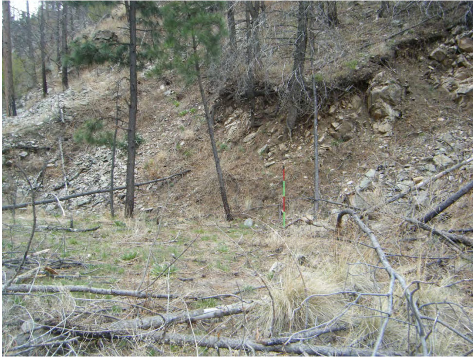
Photo 7-Looking southwest at CutPly-1.
