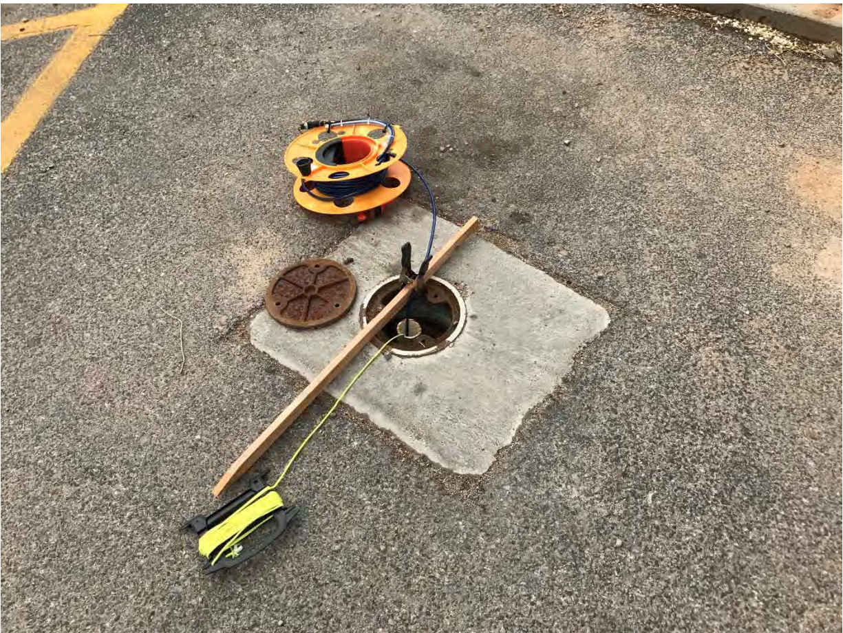
Photo 4: Monitoring well MW-17 with slug and transducer installed in well.
