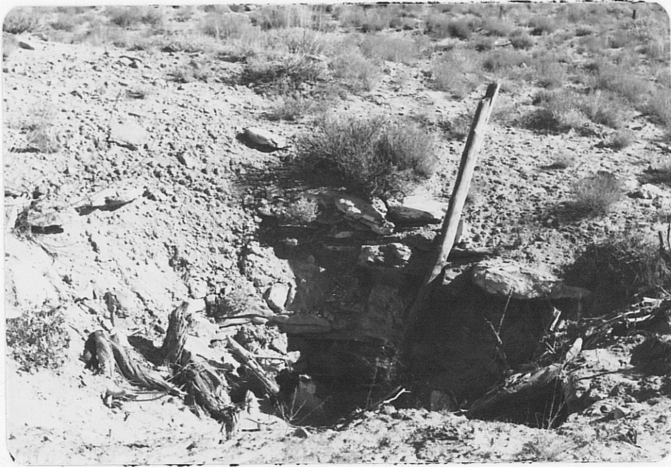
Photo (c) Ventilation shaft of Begay #1; pole at right is 5" diam, 7' long.
