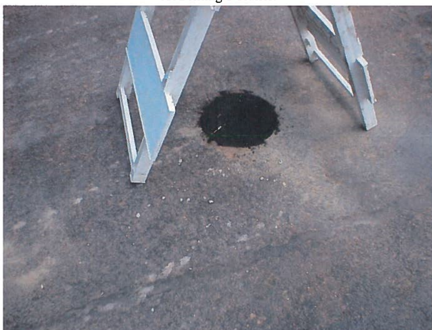
Photo 4 V-1 plugged and abandoned.
