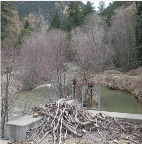
Current South Ditch Diversion structure.
