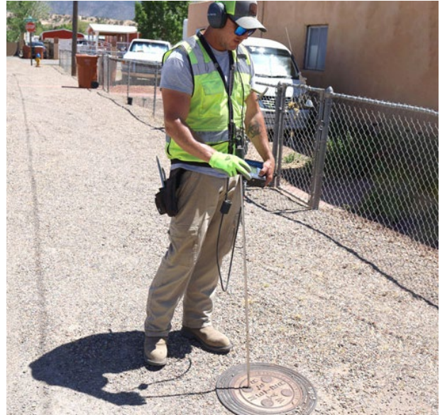
Using acoustic correlation, a survey technician verifies a leak at a satellite-identified point of interest (POI).
