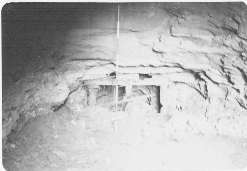
Photo (f) Drift driven NW at end of trench shown in photo (e); trench terminates in a 25' high open slope, and drift is driven into north face of slope; range pole at center for scale.
