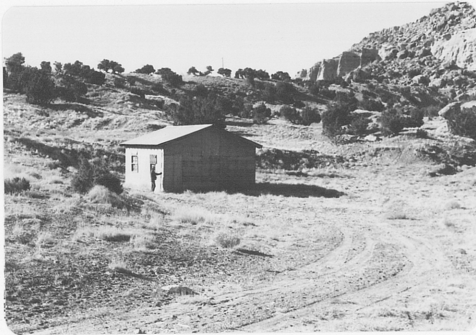
Photo (d) Metal shed about 350' southwest of shaft; note person at left side of shed for scale.
