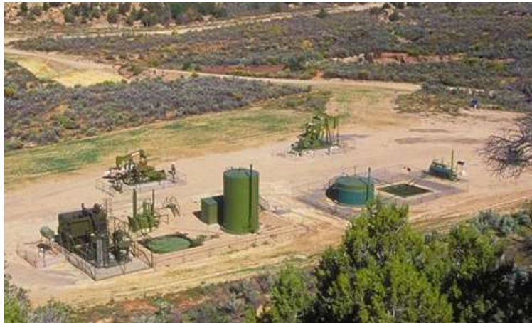
Figure 3. Example of stand-alone condensate tank at a production facility
