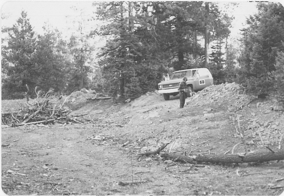
Photo (a) Bulldozer cuts-Tusas east slope.
