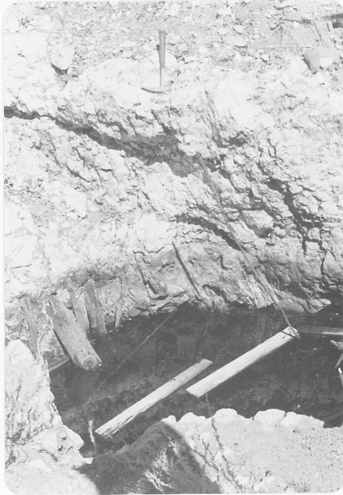
Photo (b) Close up of the small, water filled shaft on the La Paloma workings. Note hammer for scale.
