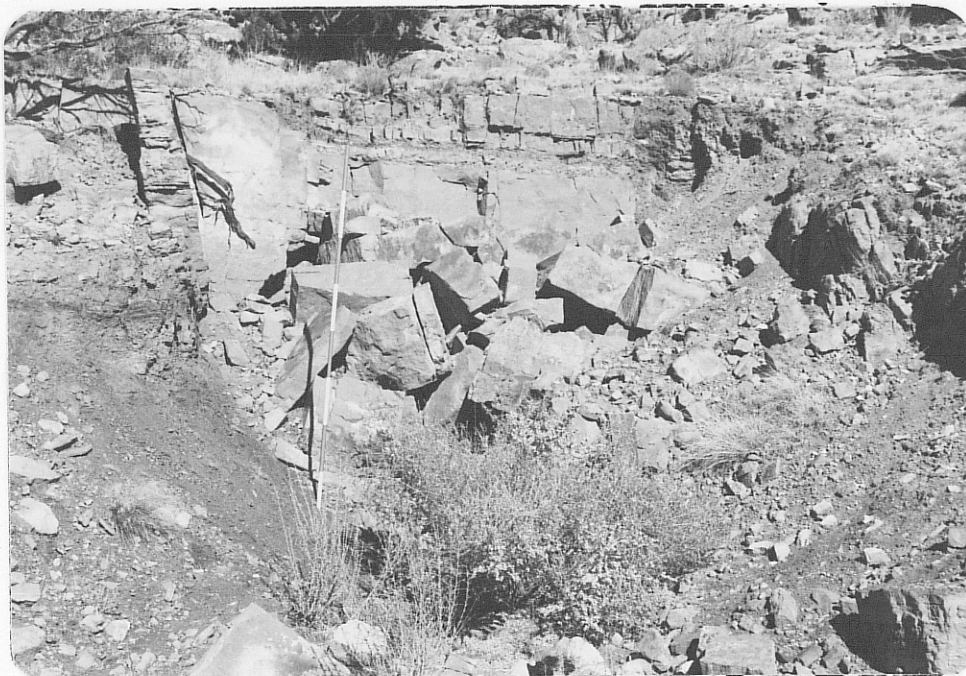
Photo (d) Looking northward at caved entrance to fourth adit (easternmost) in series of four.
