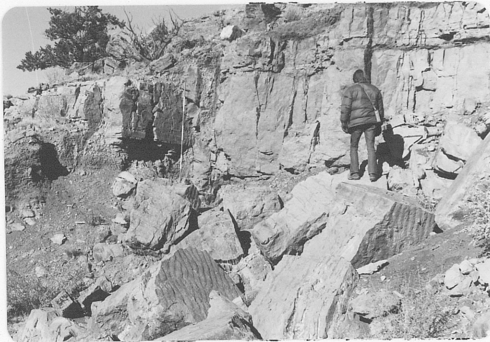
Photo (c) Looking northwestward at caved entrance to third adit in series (going eastward).
