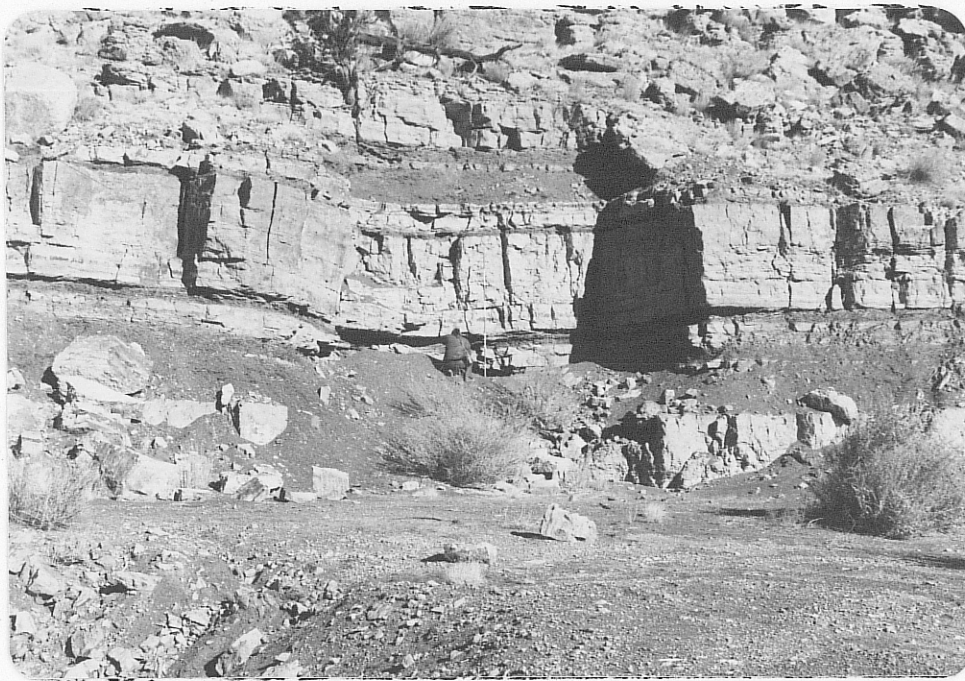
Photo (a) Looking northward at partially caved entrance to westernmost adit at the Febco Mine.
