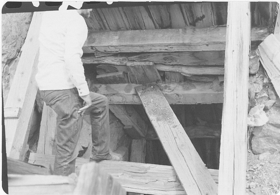
Photo (b) Close-up of opening to the Union decline.
