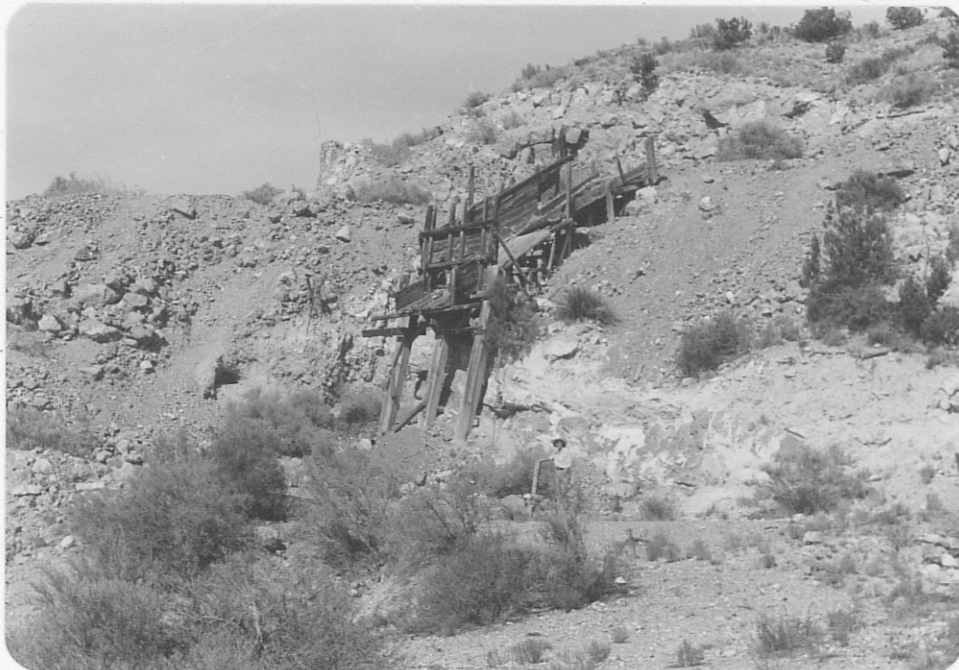
Photo (b) Looking northward at wooden ore chute and load out area at Lucky Don Mine; note person at claim marker in load out area for scale.
