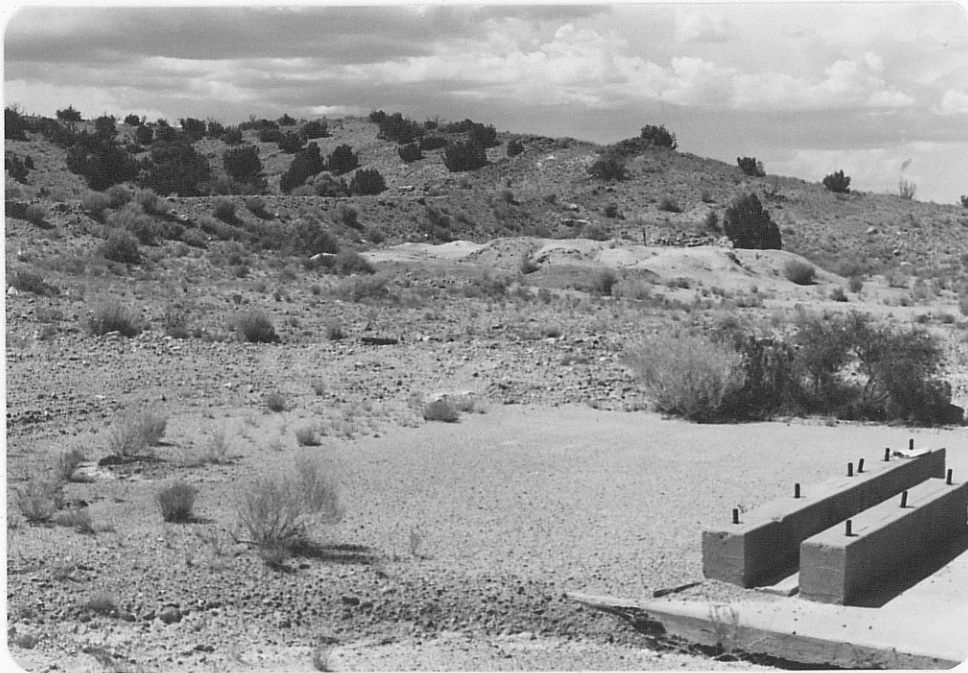
Photo D - Jeter hoist foundation and mine dump looking NW.
