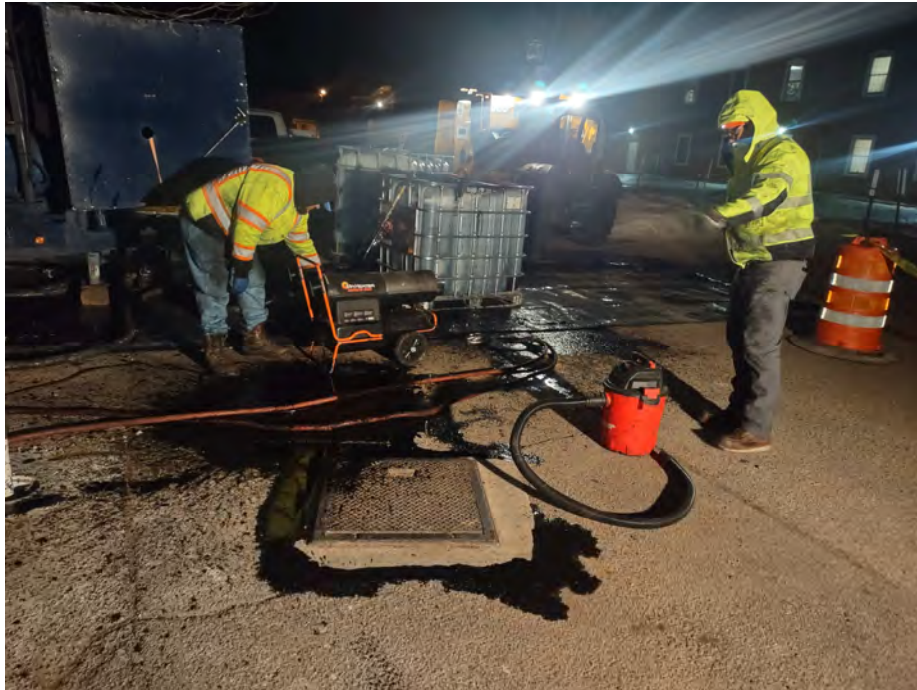
Cleanup of PetroFix® around DV-4 Using a Vacuum and Water
