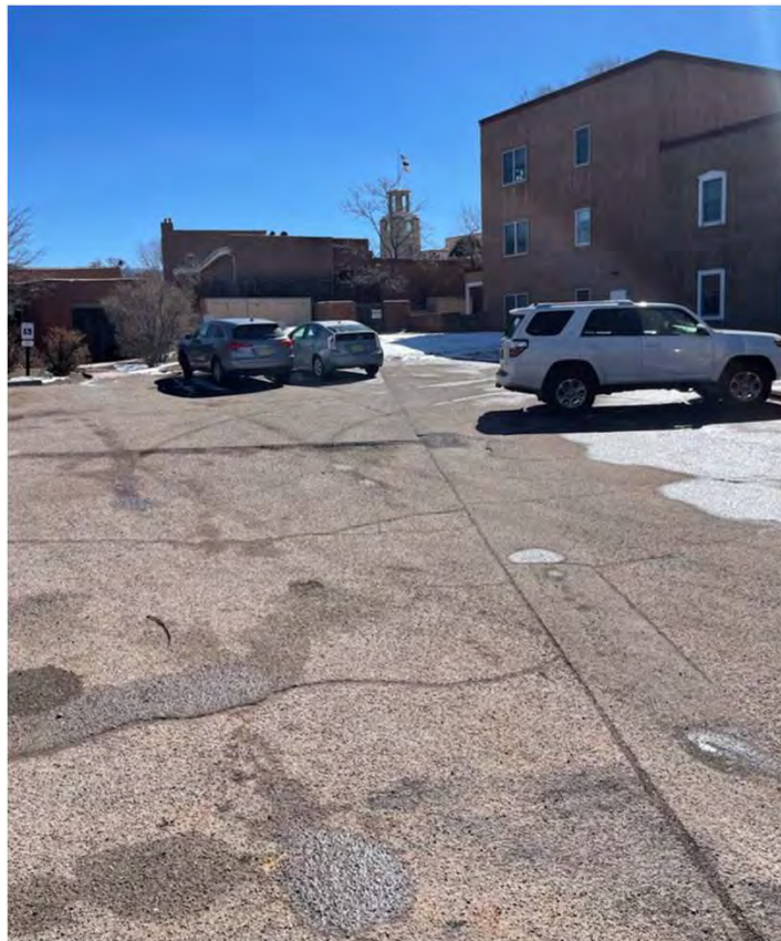
Cleaned up Surfaces before De-Mobilization
