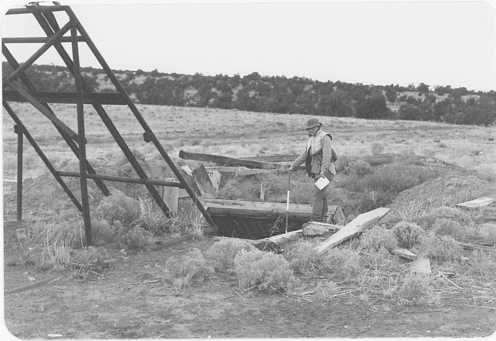
Photo (e) Close-up of headframe and inclined shaft shown in (d).
