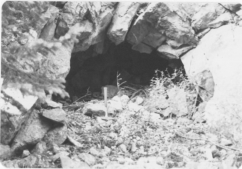
Photo (f) Beginnings of small adit east of the main dump.
