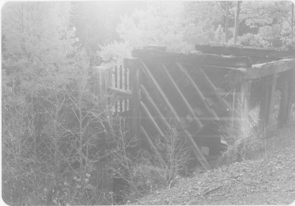
Photo (c) Stamp mill west of the Black Copper Canyon shaft.
