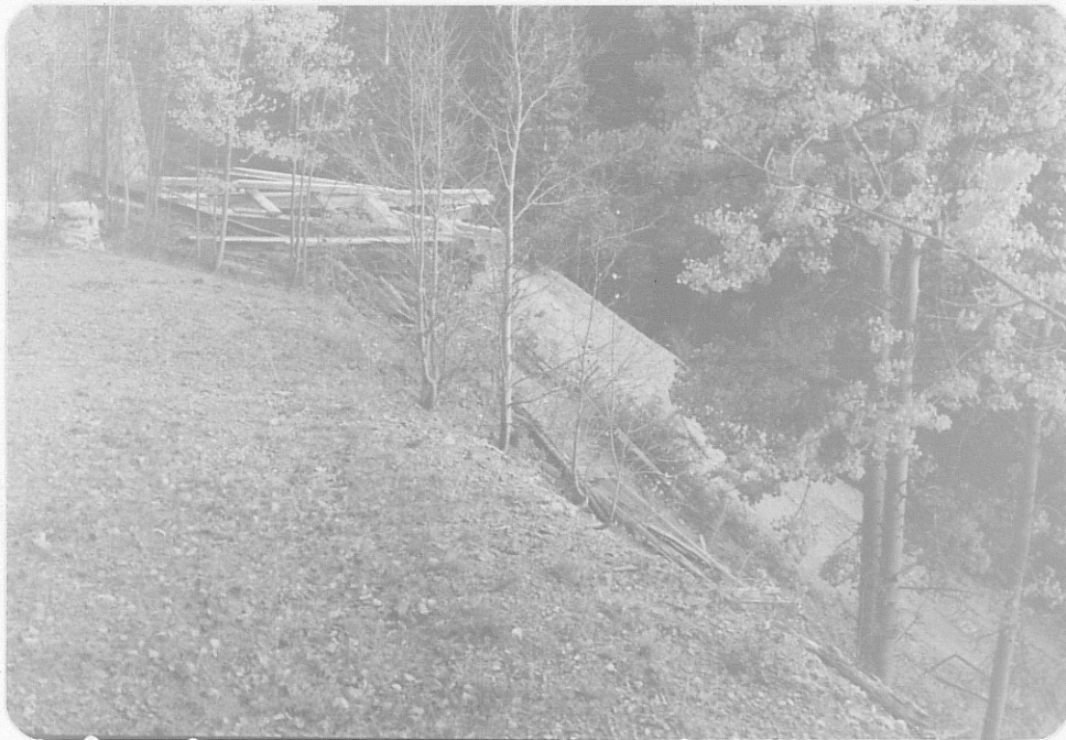
Photo (a) Collapsed shaft at Black Copper Canyon.
