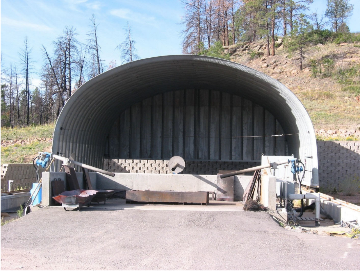
Figure 1-2 Photograph of Technical Area 16- 388 (TA-16-388) Flash Pad
