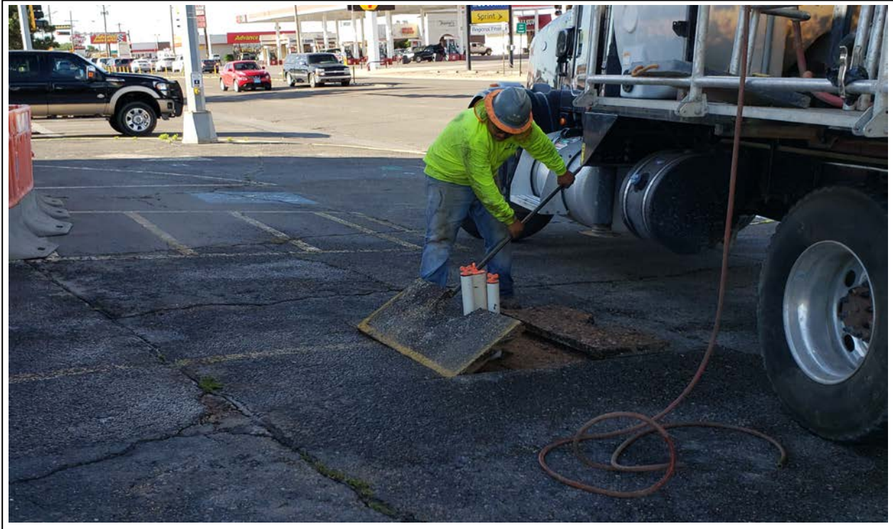
13. Removing asphalt for the RW-2 well pad completion (view to north)
