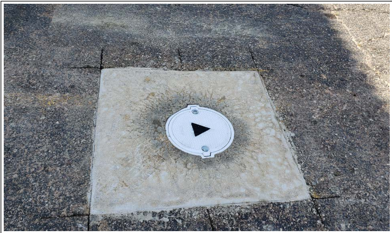
14. Well pad and vault completion at RW-2 (view to west)
