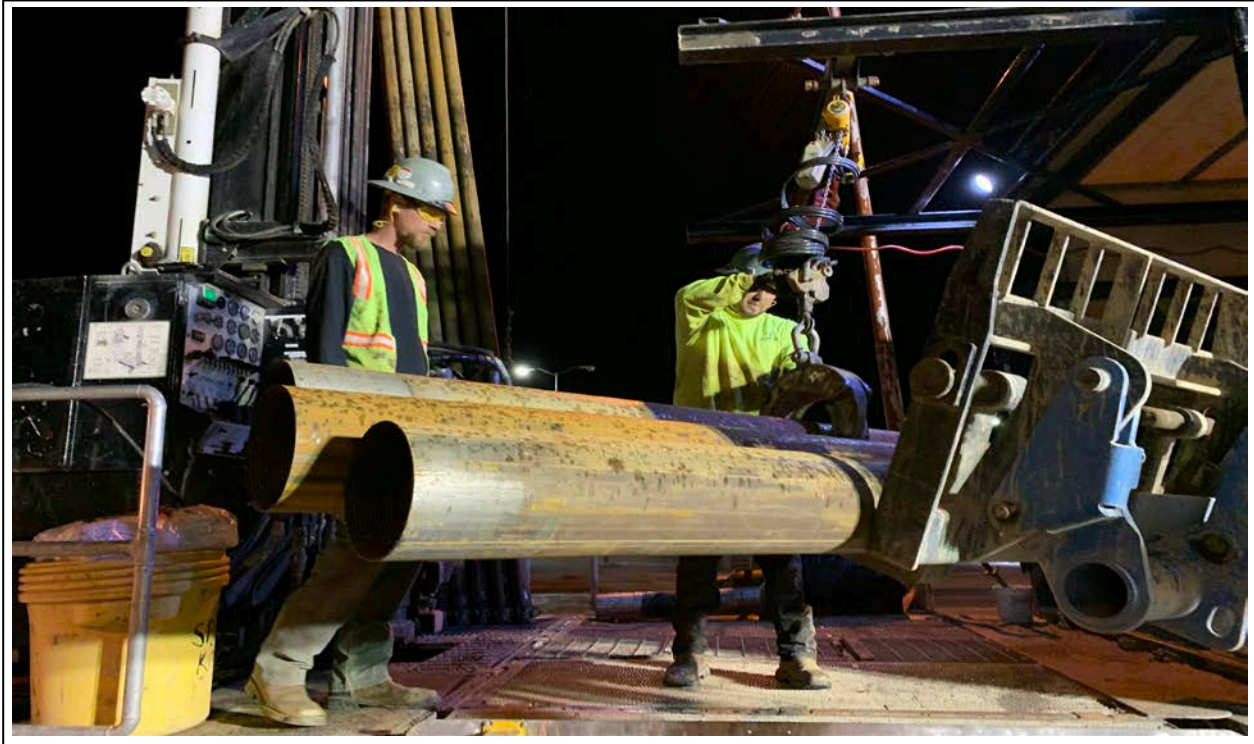
9. Moving sonic casing during night shift drilling of RW-2 (view to east)
