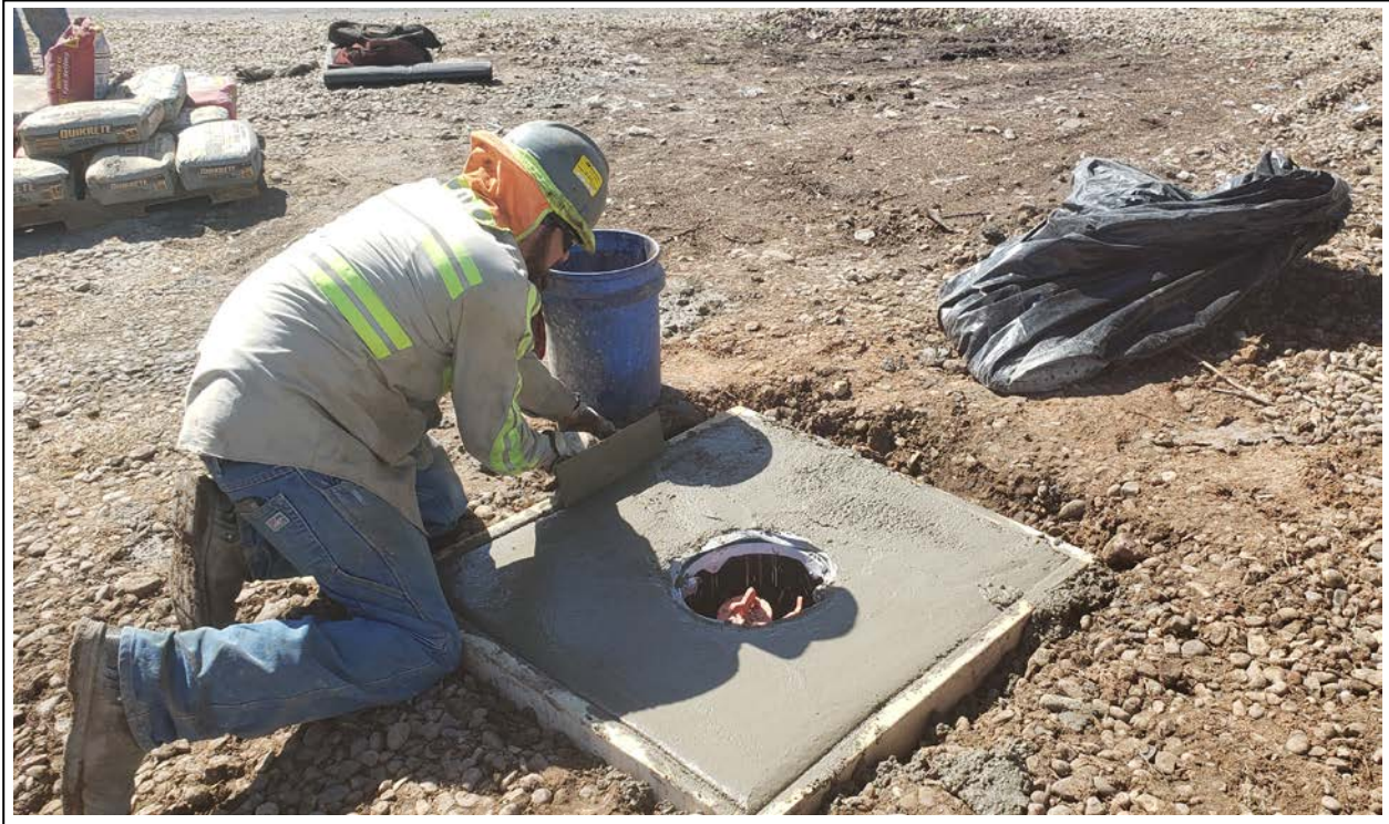
21. Well pad during installation at RW-1 (view to northwest)
