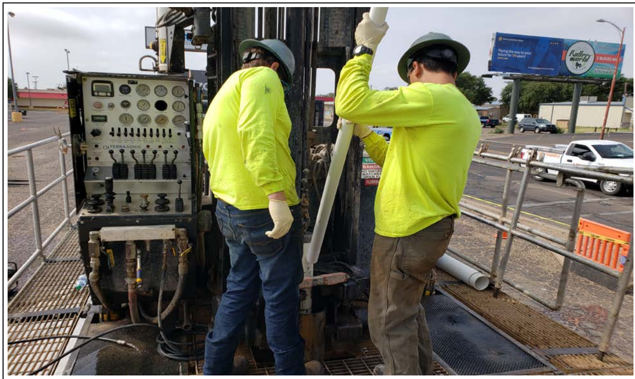
34. Installation of 2-inch screen for RW-3 (view to south)
