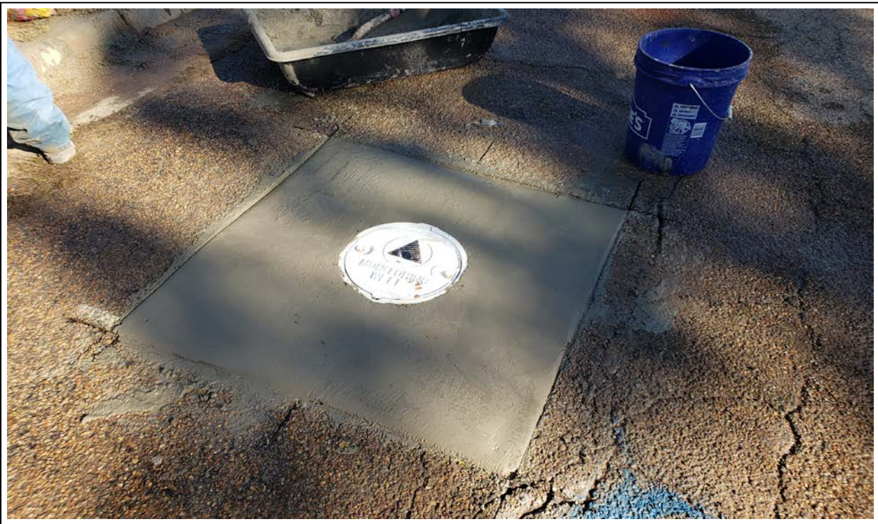
44. Well pad and vault completion at MW-14 (view to northwest)
