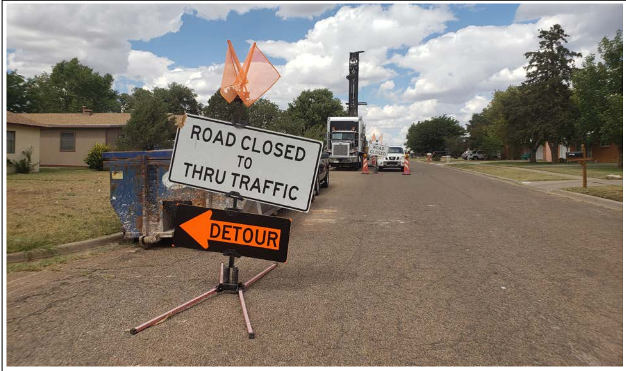
41. Traffic control for MW-14 (view to north on N. Lea Street)
