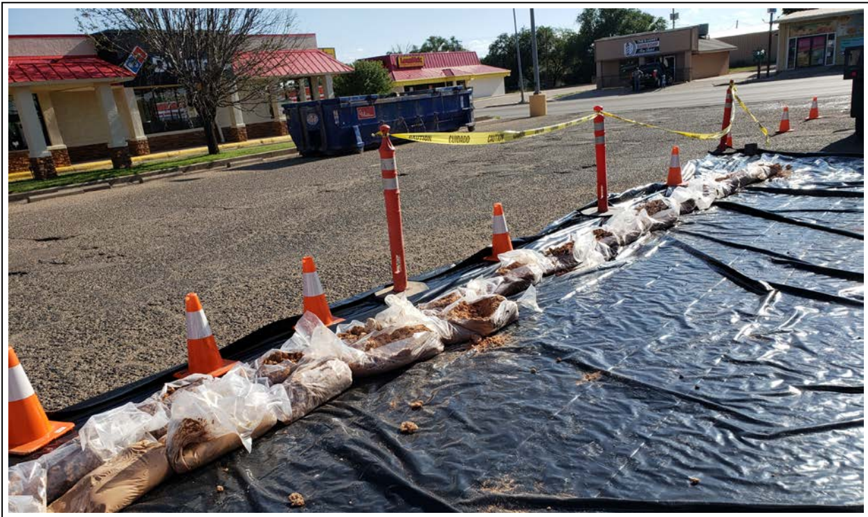
26. Sonic core cuttings for BW-7R and mud box placement (view to southwest)
