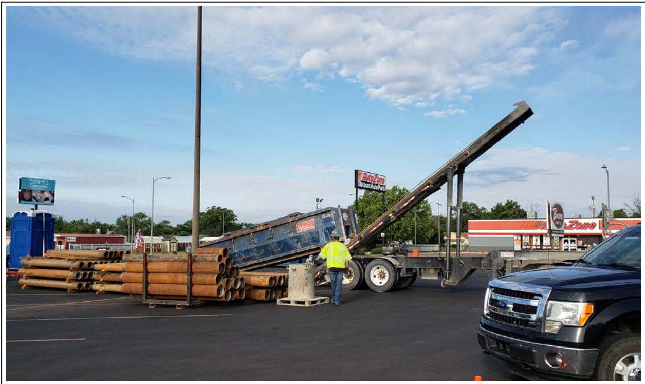
2. Mud box delivery (view to southwest)
