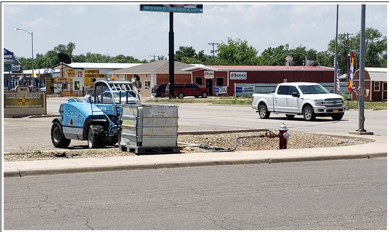
4. Filling water tank from the city hydrant (view to southwest)
