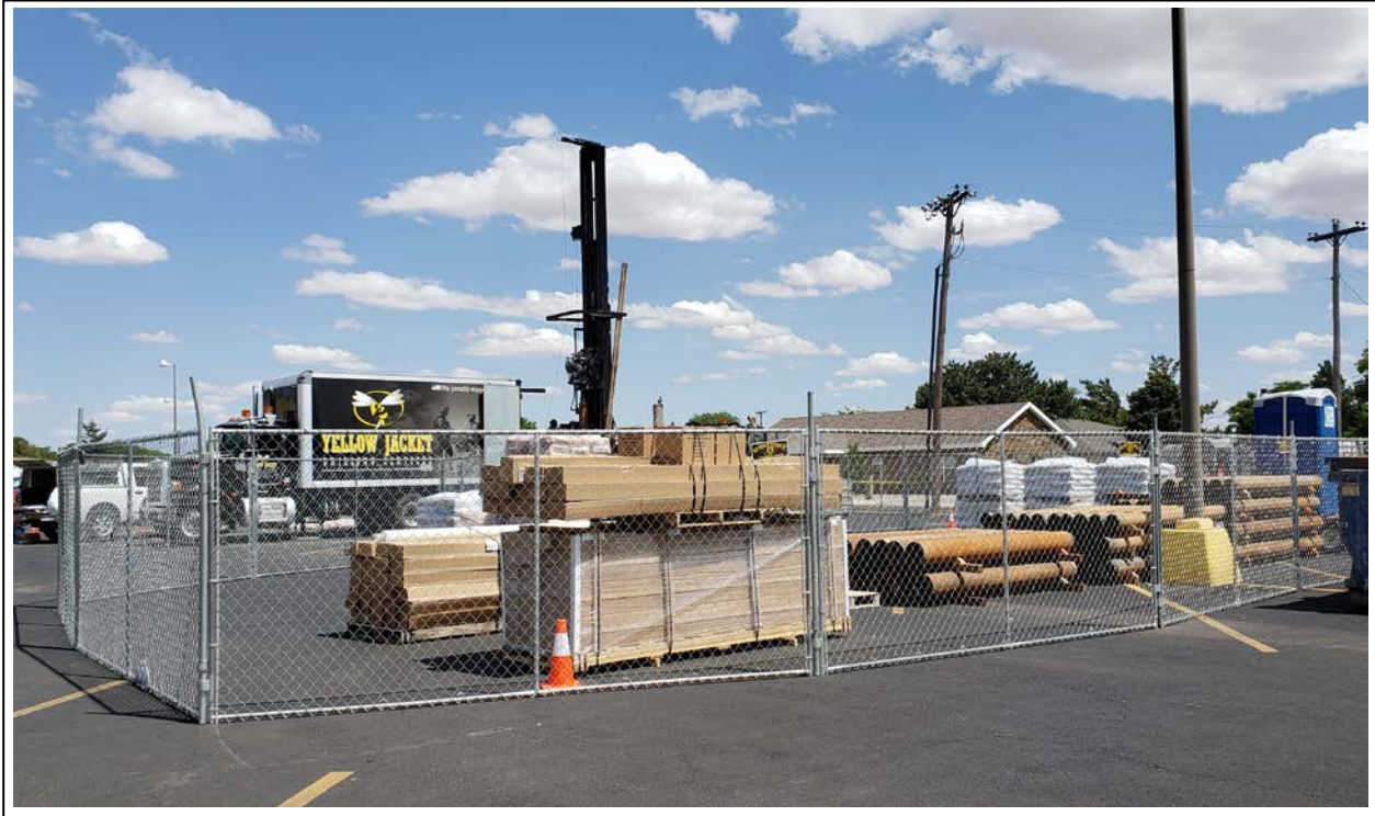
3. Drilling and well construction materials in the laydown yard (view to southeast)
