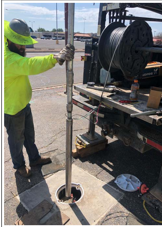
49. Installation of the development pump at RW-2
