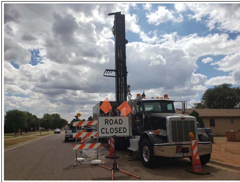
42. Traffic control for MW-14 (view to south on N. Lea Street)
