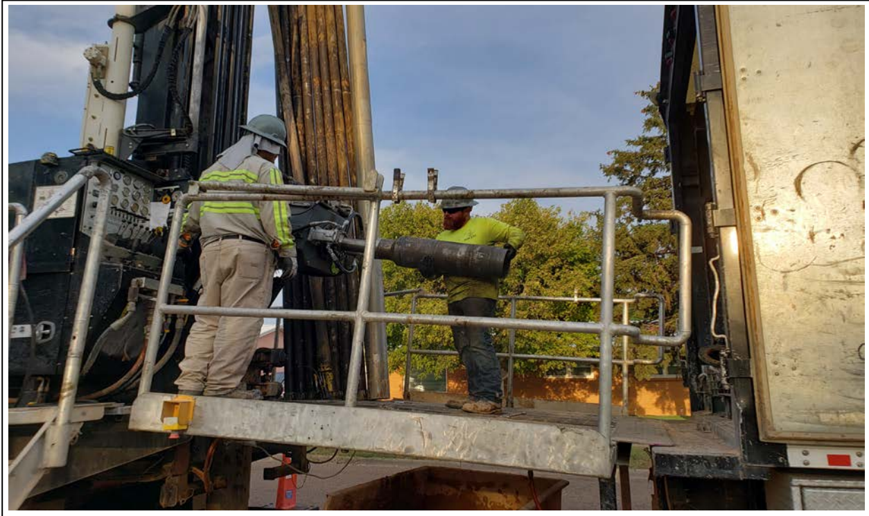
39. Preparing to remove sonic casing at MW-14 (view to west)
