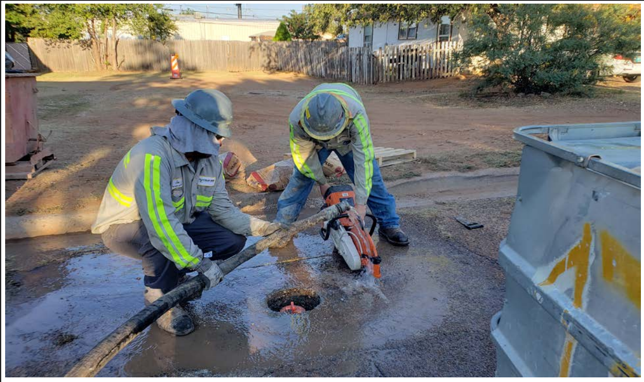
43. Saw-cutting asphalt for well pad at MW-14 (view to west)
