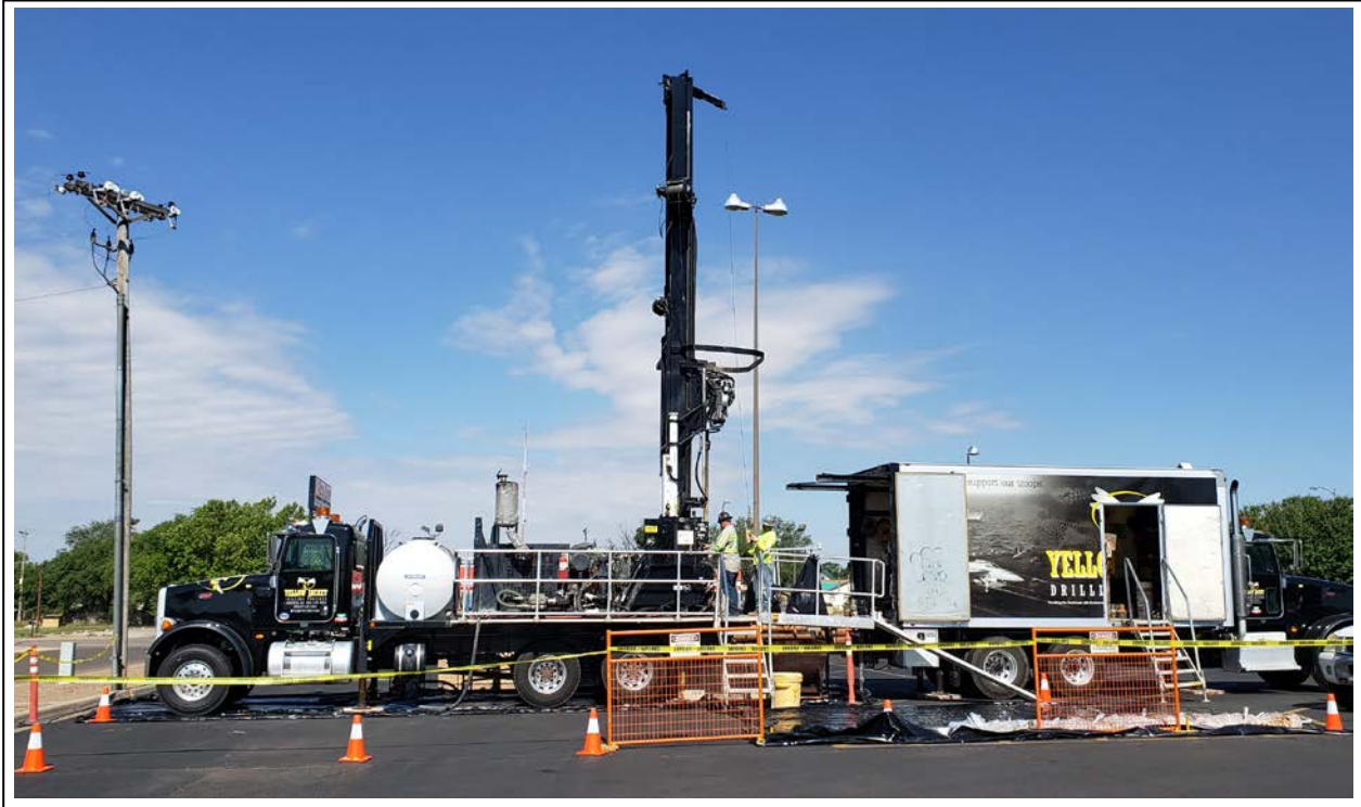
1. Drill rig set up for monitor well MW-11 (view to west)
