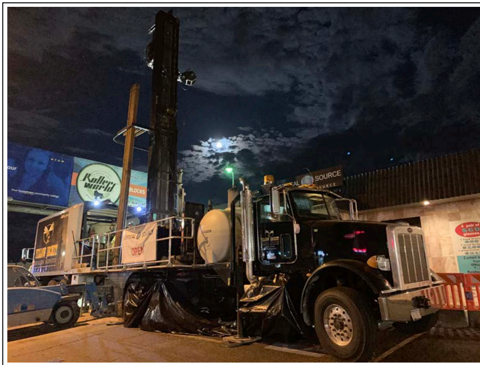
10. Overnight drilling at RW-2 (view to southwest)
