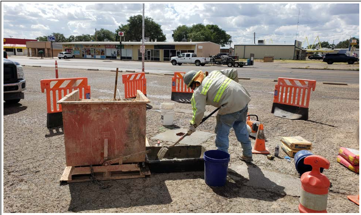
36. Mixing concrete for the well pad at RW-4 (view to southwest)
