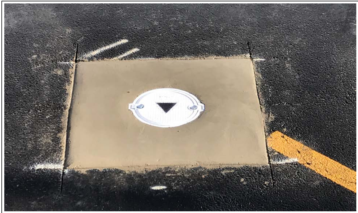
6. MW-11 well pad and vault completion (view to south)
