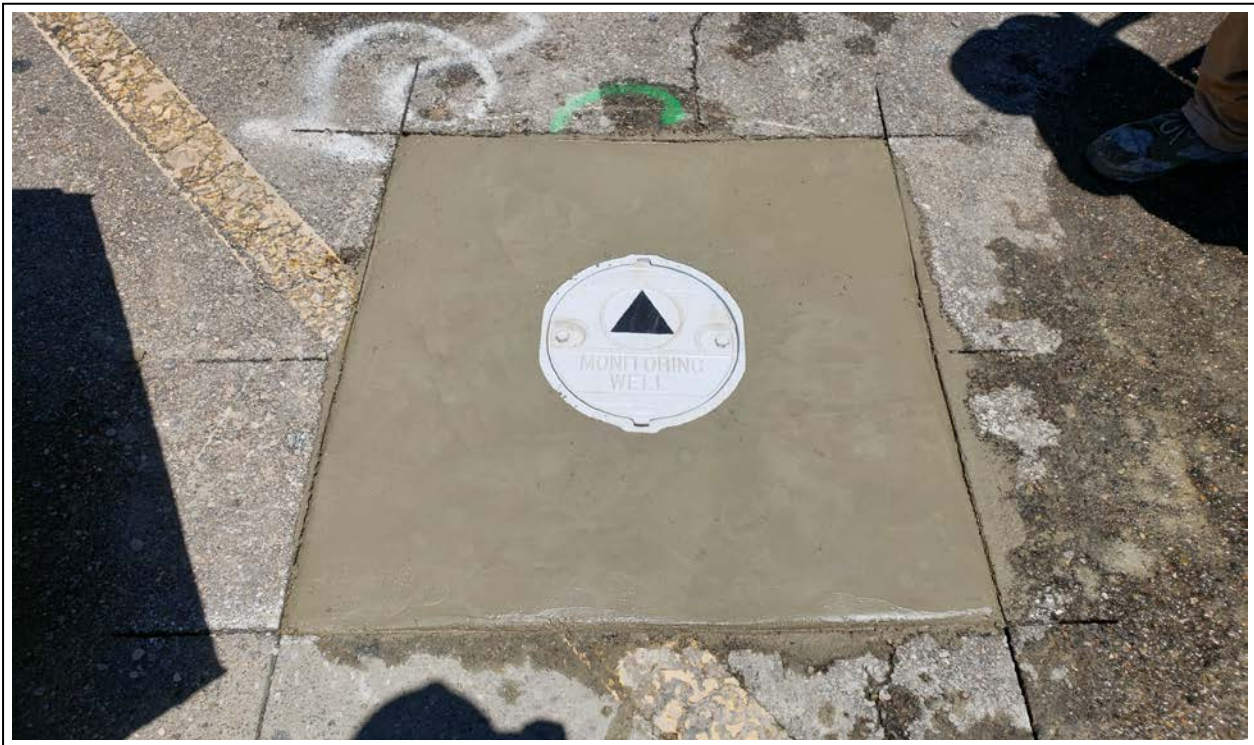
24. Well pad and vault completion at MW-12(view to north)
