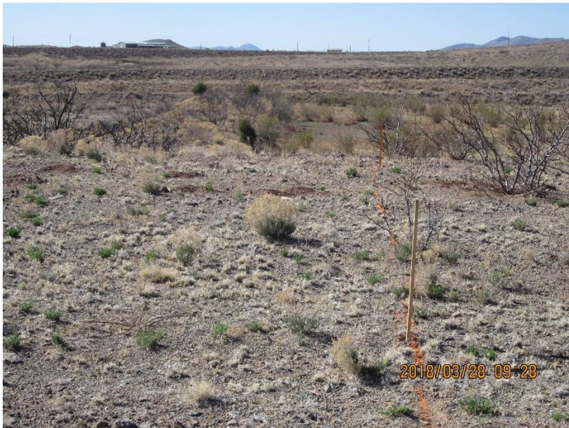
Figure 2: Excavation Centerline Staking Looking from Top of Dike South into South Cell (2018-03-28)
