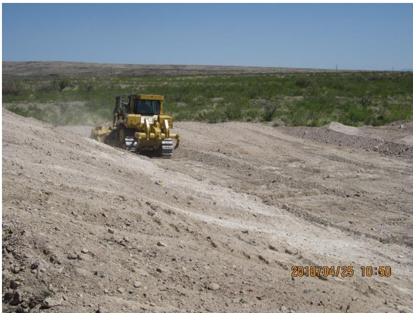
Figure 8: Regrading of North Side of Breach Weir (2018-04-25)
