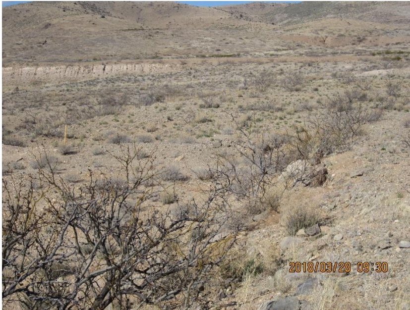
Figure 3: Excavation Centerline Staking Looking West from Top of Dike (2018-03-28)
