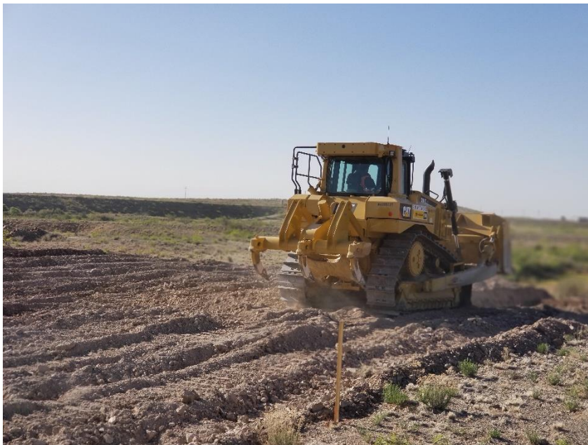
Figure 4: Breach Excavation Start (2018-04-19)
