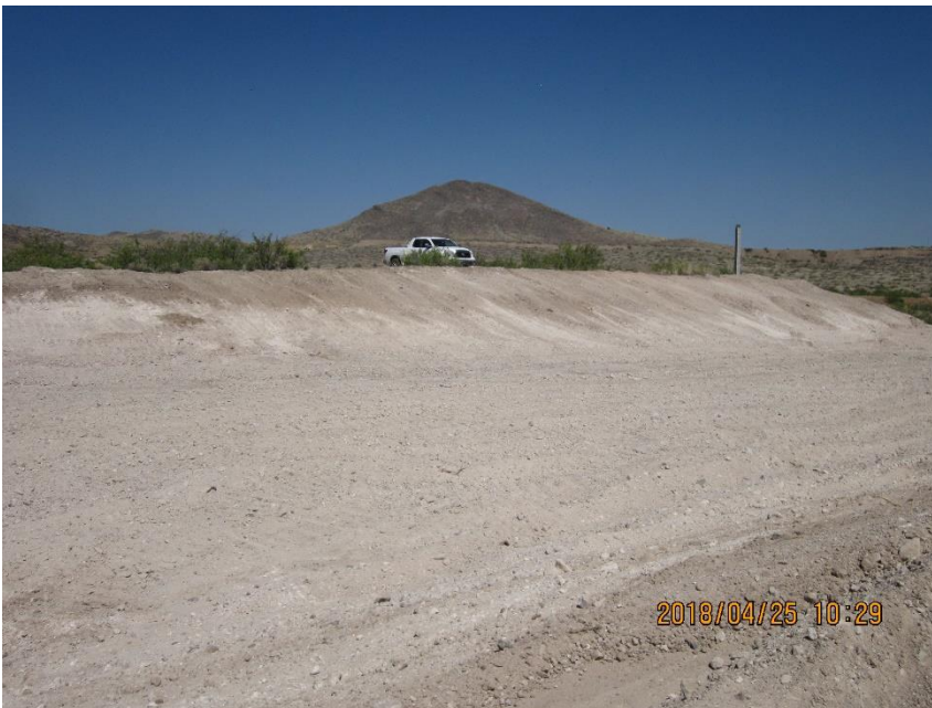
Figure 6: At SE Weir Crest Looking Northwest (2018-04-25)
