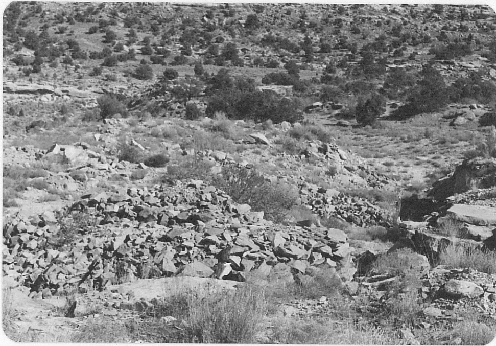
Photo (a) Looking E SE into open cut of King #2. Note access.
