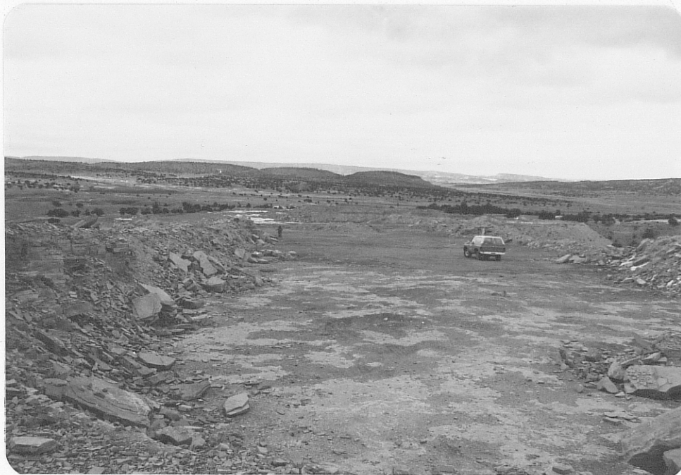
Photo (b) Looking northeastward from southern edge of workings shown in photo (a). Stripped area extends for 600' to 800' into distance.
