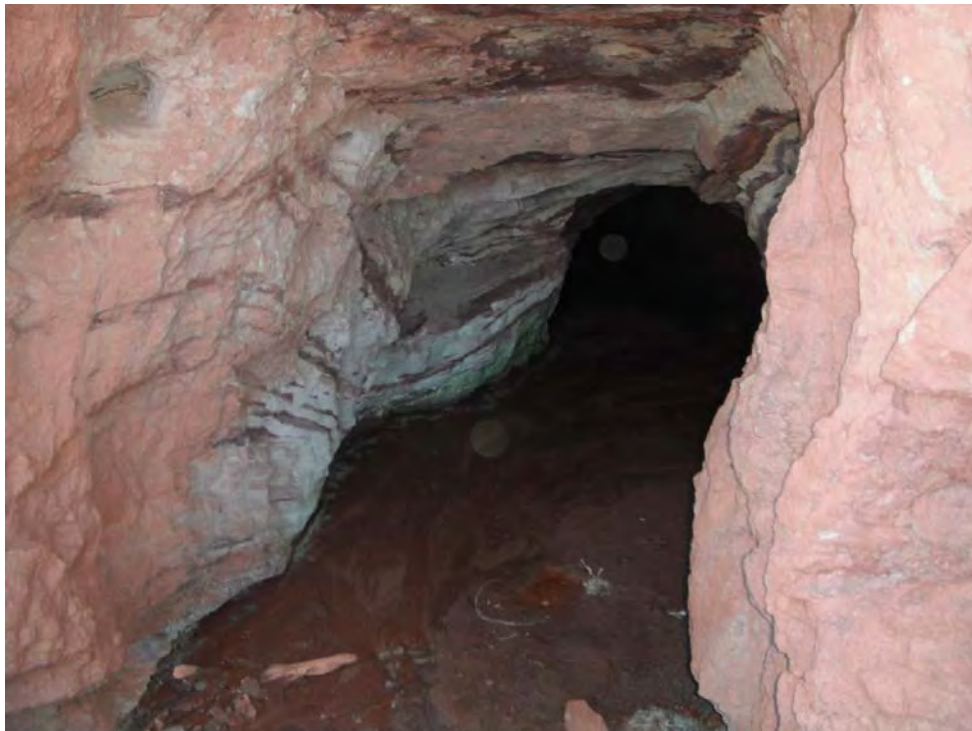
Photo 6-Looking east at wall of Adit-1.
