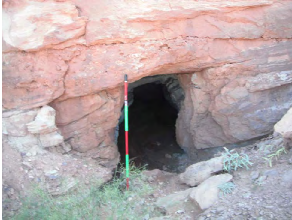
Photo 5-Looking east at Adit-1.
