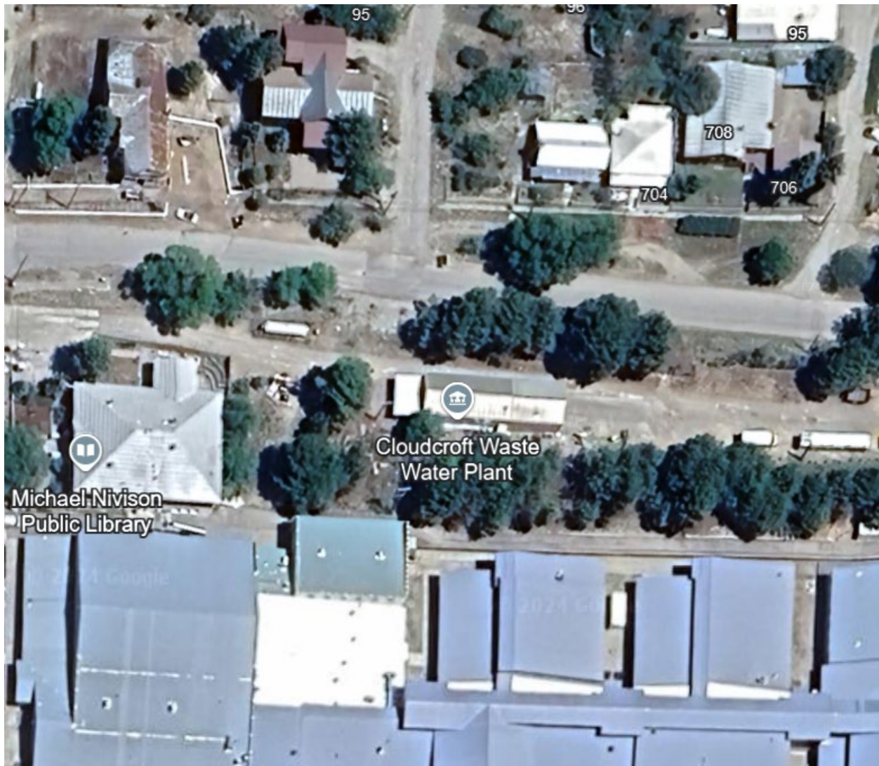
Aerial View of the Cloudcroft Wastewater Treatment Plant (Source: Google Earth)
