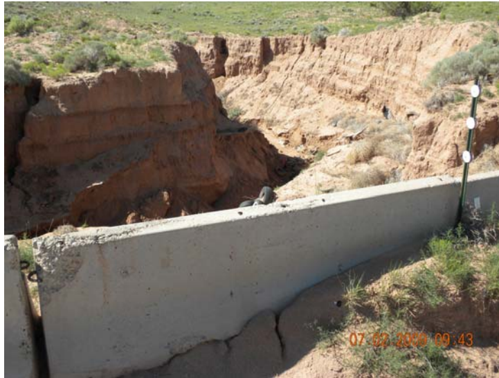
P1: Roundy Manol Strip excavation
