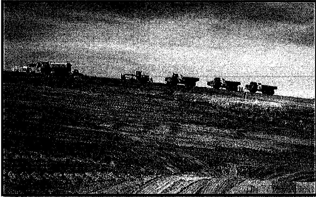
Repository Construction in October 2012
