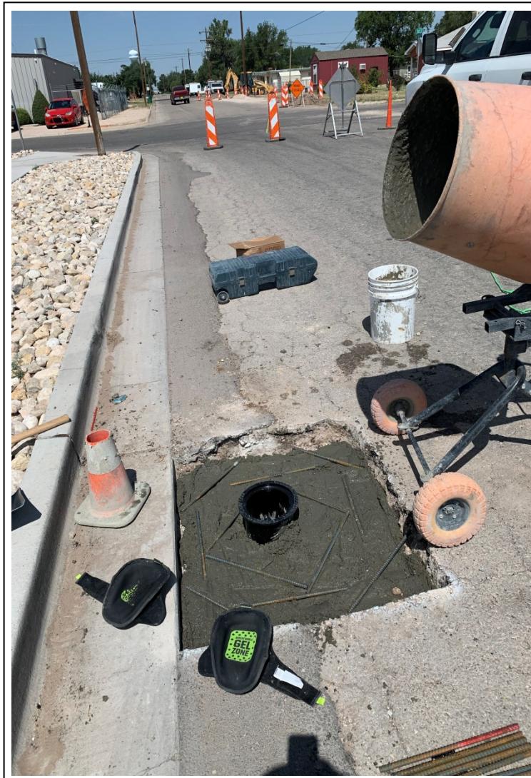
3. New vault and re-bar reinforced well pad installed around existing well W-7.
