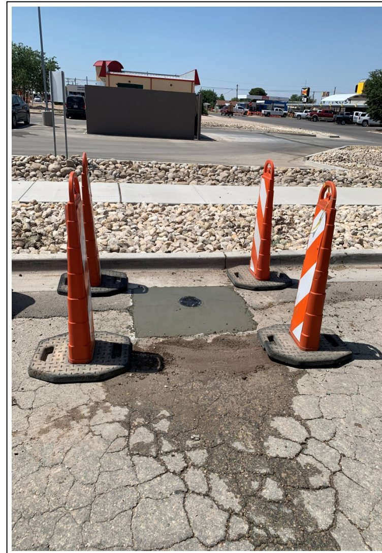
4. Finished well vault and pad at well W-7, view to the south.
