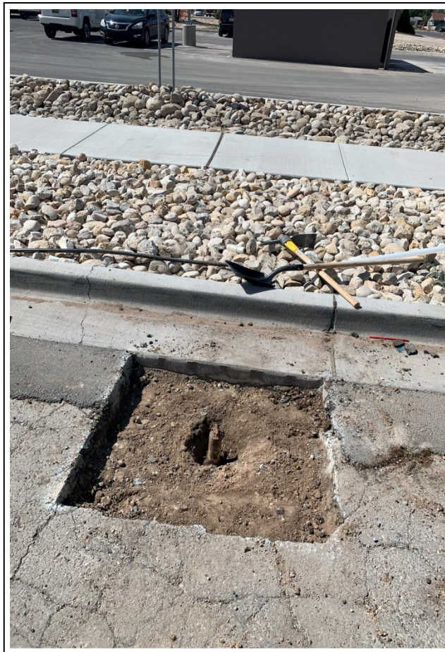
2. W-7 wellhead excavated and surrounding asphalt saw-cut, view to the west-northwest.
