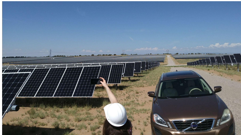
50MW Encino solar farm in NM
