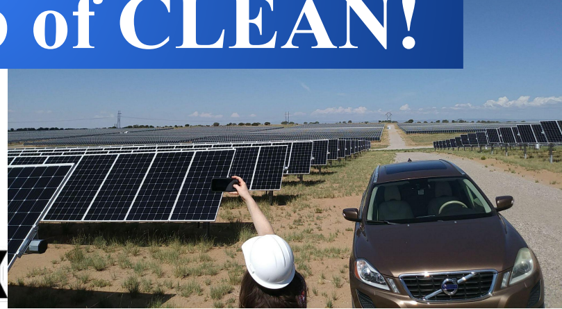
50MW Encino solar farm in NM
