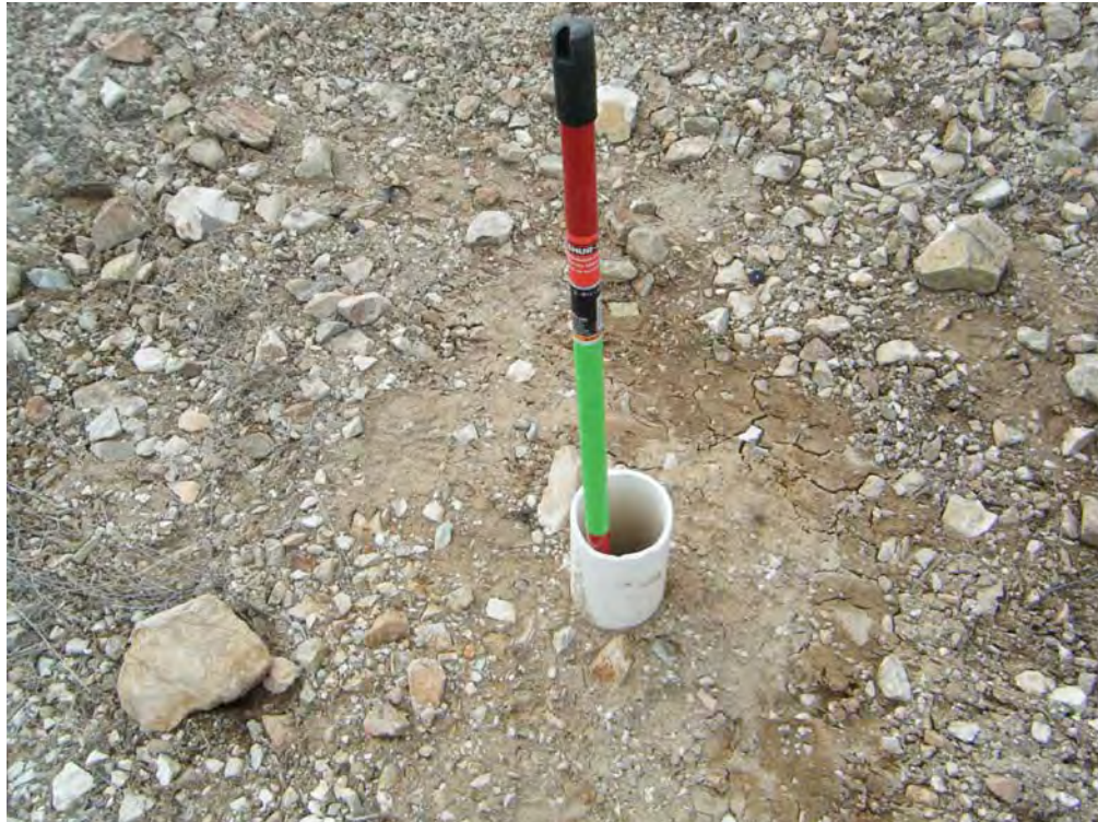
Photo 9 – Closeup of vent pipe in Photo 8 (LU-1).
