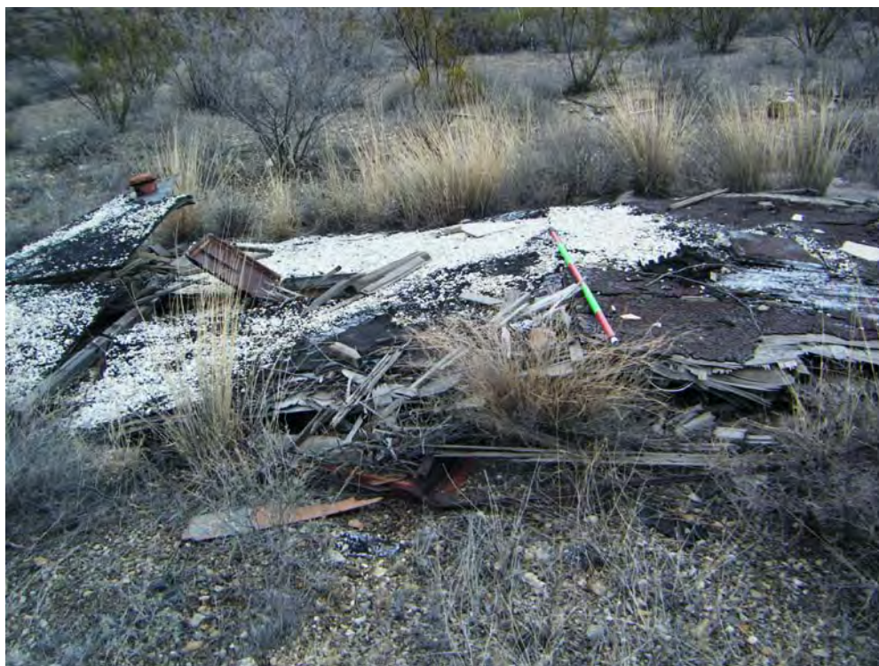
Photo 48 – This collapsed structure (StrucPly-1) may be the trailer house mentioned in the Anderson Report.
