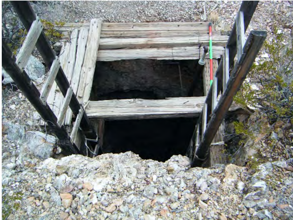
Photo 39 –Looking southeast at Shaft-5, replicating photo (h) in the Anderson report.
