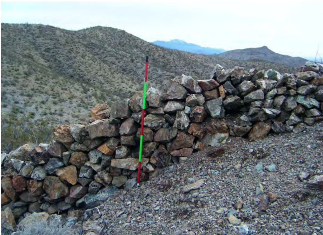
Photo 29 – Side view of load out ramp, looking southeast (Loadply-1).
