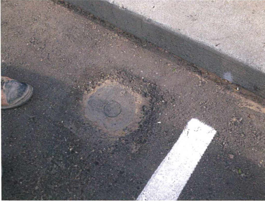
Photograph No. 29 Well W-37 partially paved over, pre-abandonment.
