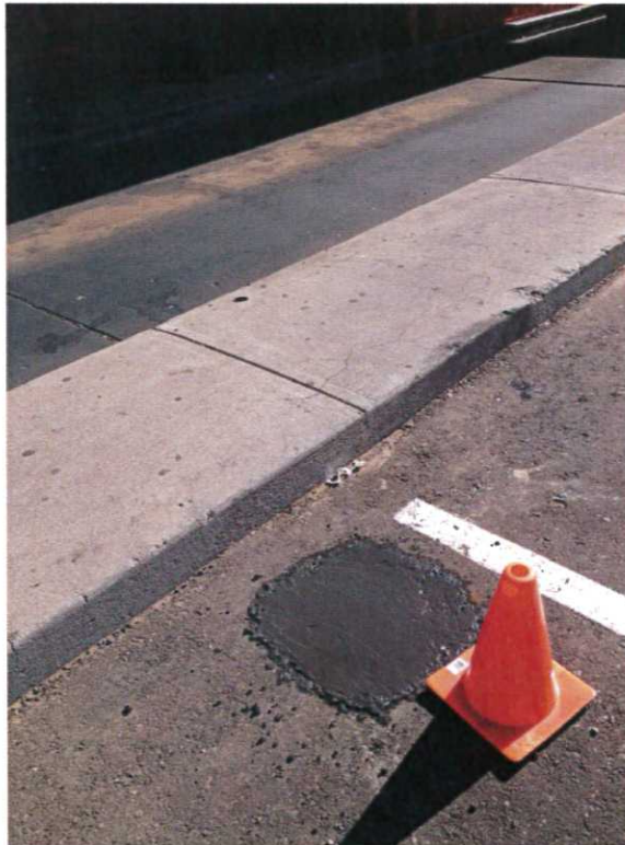
Photograph No. 30 Well W-37 post abandonment.
