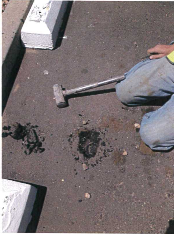
Photograph No. 25 Locating Well W-35 under asphalt.
