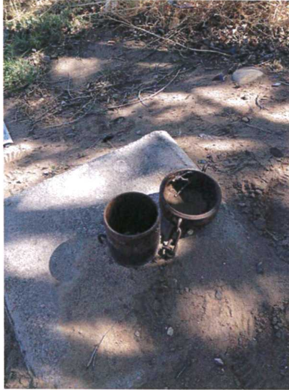
Photograph No. 1 Well MW-1 pre-abandonment.
