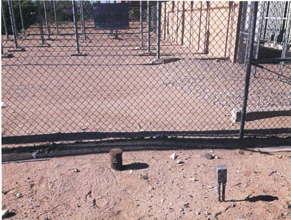
Photograph No. 17 Well MW-6 pre-abandonment.
