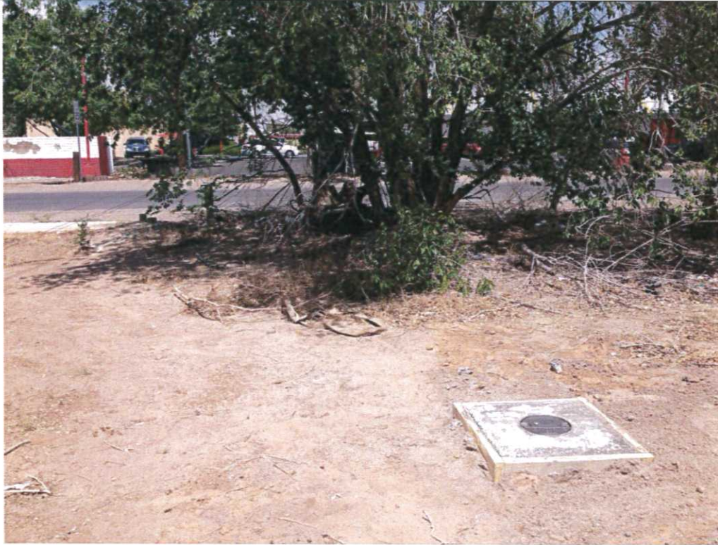
Photograph No. 7 Completed replacement groundwater monitoring well MW-1R.
