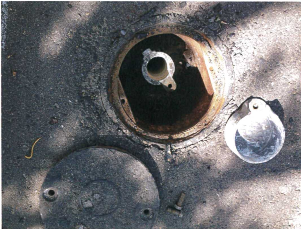
Photograph No. 28 Well W-36 opened.
