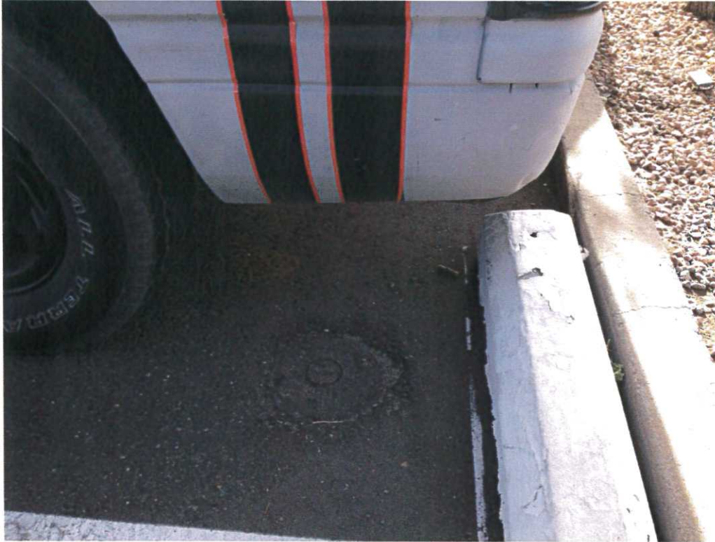
Photograph No. 27 Well W-36 partially paved over.
