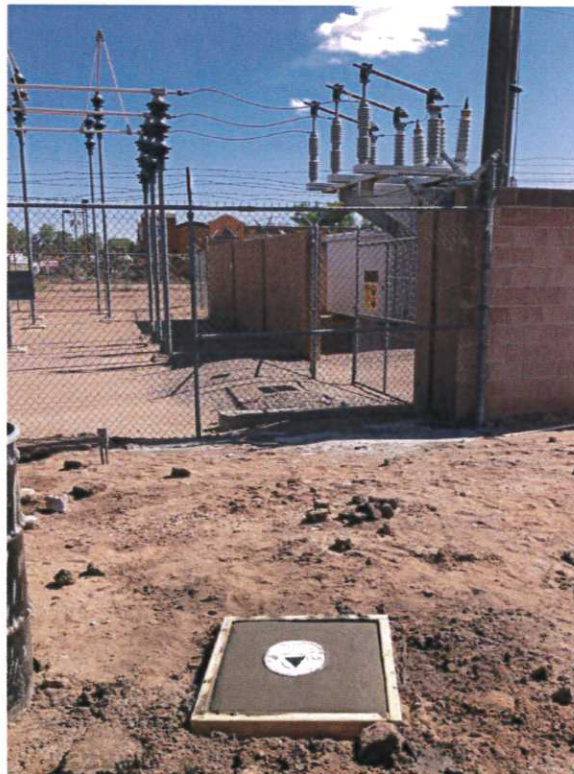
Photograph No. 18 Replacement well MW-6R with area of well MW-6 post abandonment (middle left).
