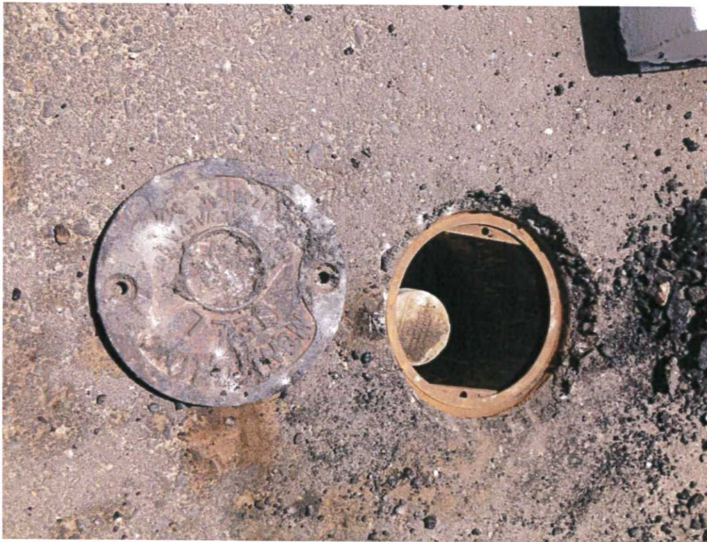
Photograph No. 26 Well W-35 exposed and opened.
