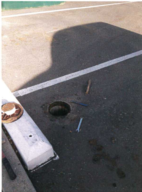
Photograph No. 24 Well W-34 pre-abandonment.
