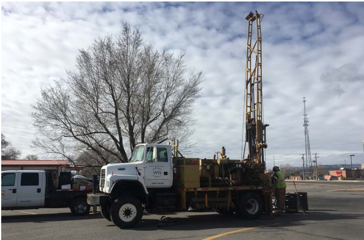
Photo 4 - Drilling MW-27, view to southwest
