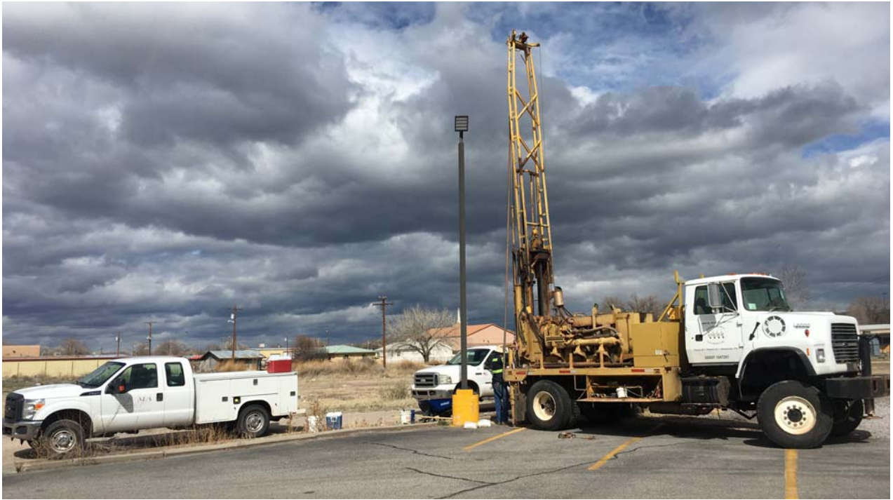
Photo 3 - Drilling MW-26, view to northeast
