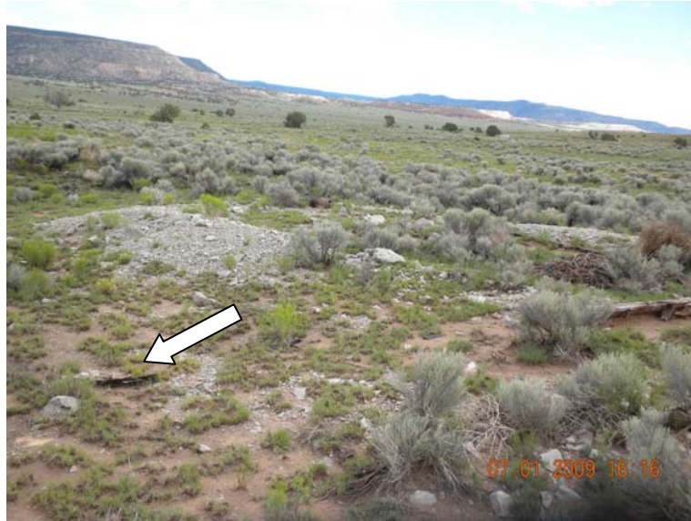
P2: Barbara J #3 Mine shaft covered by rusted steel plate (arrow)
