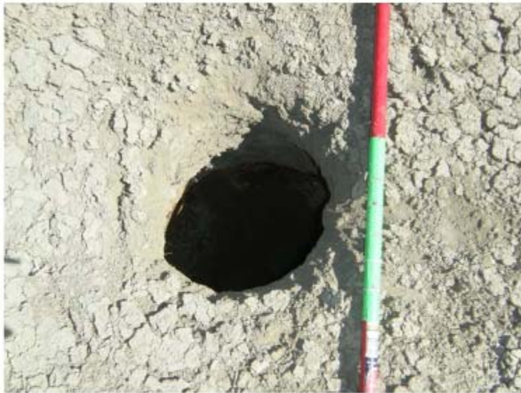
Photo 4-A vent shaft (MiscPt-1) in DistPly-1.
