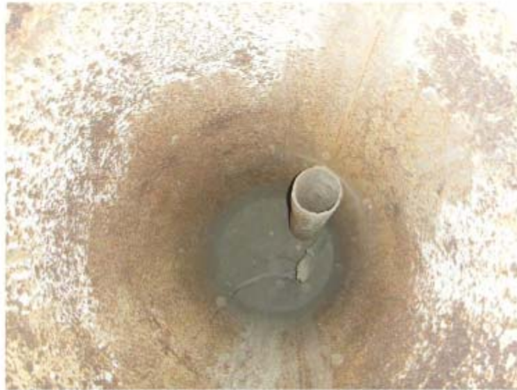
Photo 5-View down vent shaft (MiscPt-1).
