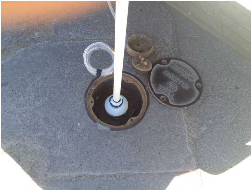
Photo 3: Walstad SVE pretest production well setup
