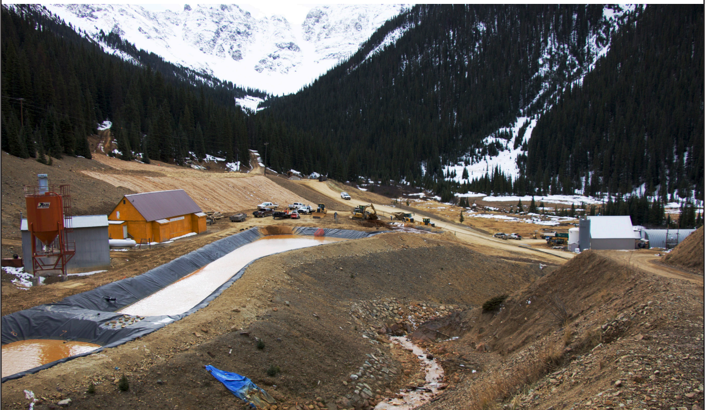
From left to right: the retired Goldfields, Inc. treatment facility, the Gold King settling ponds, and the Gladstone Water Treatment Plant.
