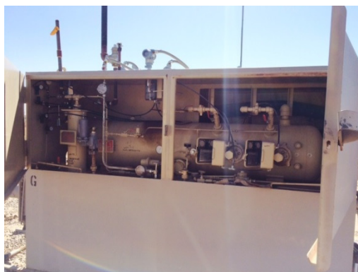
Figure 17-1 Picture of Equipment Building
