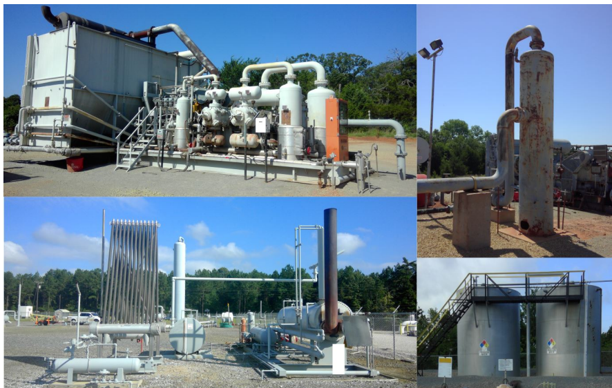
Figure 1: Typical equipment found on gathering stations. Clockwise from top left: Compressor, separator, liquid storage tanks and dehydrator.
