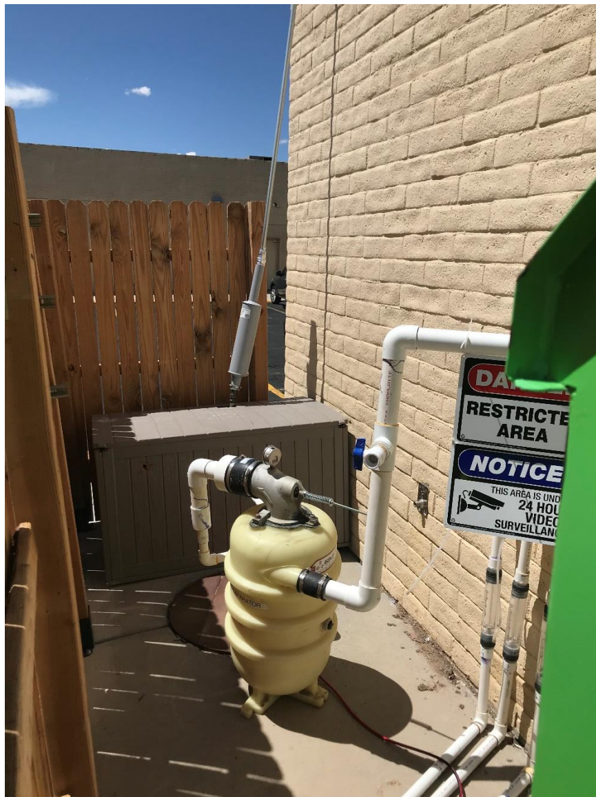
Description: Completed surface completion of nested SVE wells, SVE-1 through SVE-4.
