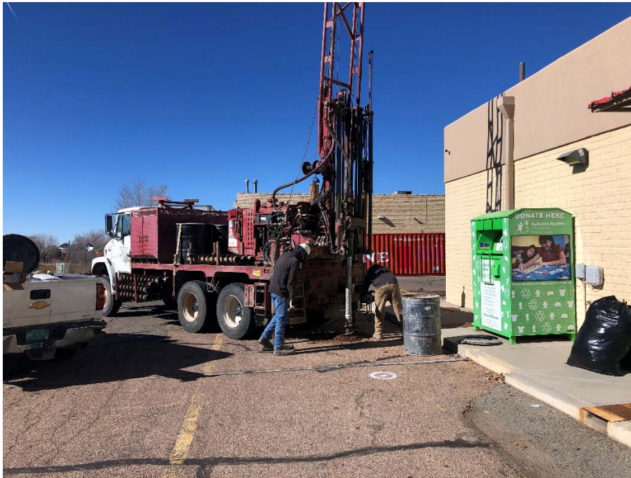
Description: Set up to drill SB-1 where SVE-1 through SVE-4 will be installed. Direction: West
