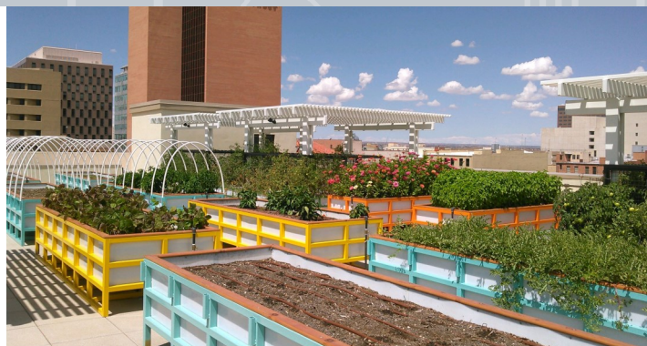
With the appropriate resources to evaluate and clean up orphan sites, many can be transformed back into economically productive properties. One example is the Imperial Building in downtown Albuquerque, complete with a rooftop garden, shown here.
