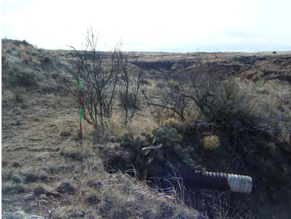
Photo 24-A culvert (MiscPt-1) in mine road Rd-2.
