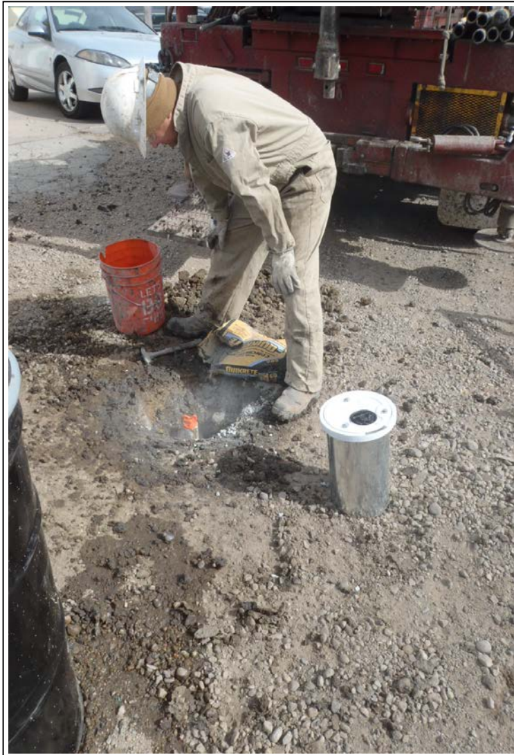
3. Monitor well AEE-1R well vault prior to completion (view to the west)
