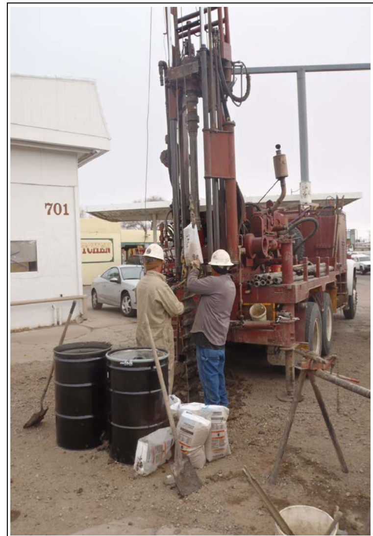
2. Monitor well AEE-1R construction (view to the northeast)
