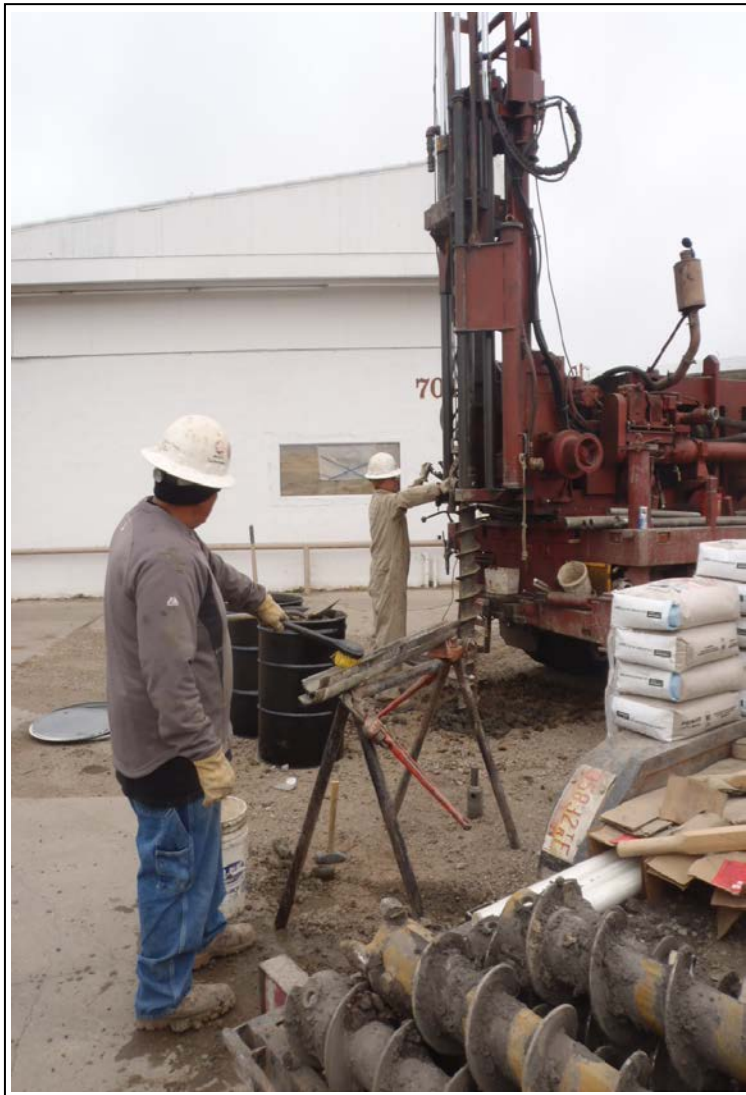
1. Drilling monitor well AEE-1R (view to the north)
