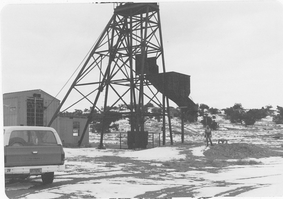
Photo (b) Close up of head frame, showing the skip suspended over shaft at ground level, and small ore pile lying below chute where person is standing.
