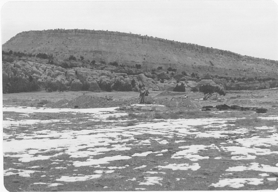
Photo (c) View to northwest of shaft and head frame, showing an extensive mine dump area that continues into the background, and an 8' x 20' concrete slab covering a small ventilation shaft and/or escapeway; person is standing on concrete slab.
