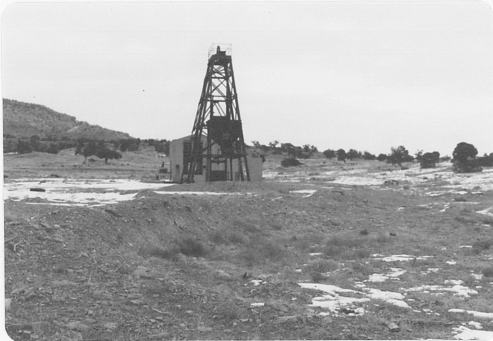
Photo (a) Looking north at head frame and hoisting shed at Sec. 25 shaft; note small dump area in foreground. Shaft is about 35' high.
