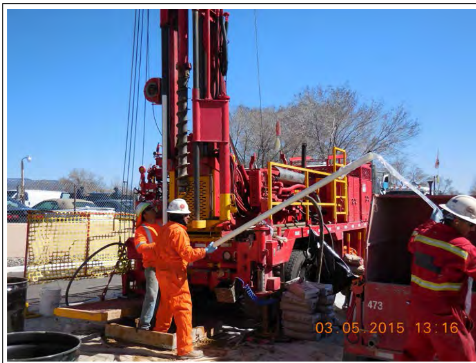
15. Installation of well casing at MW-11.
