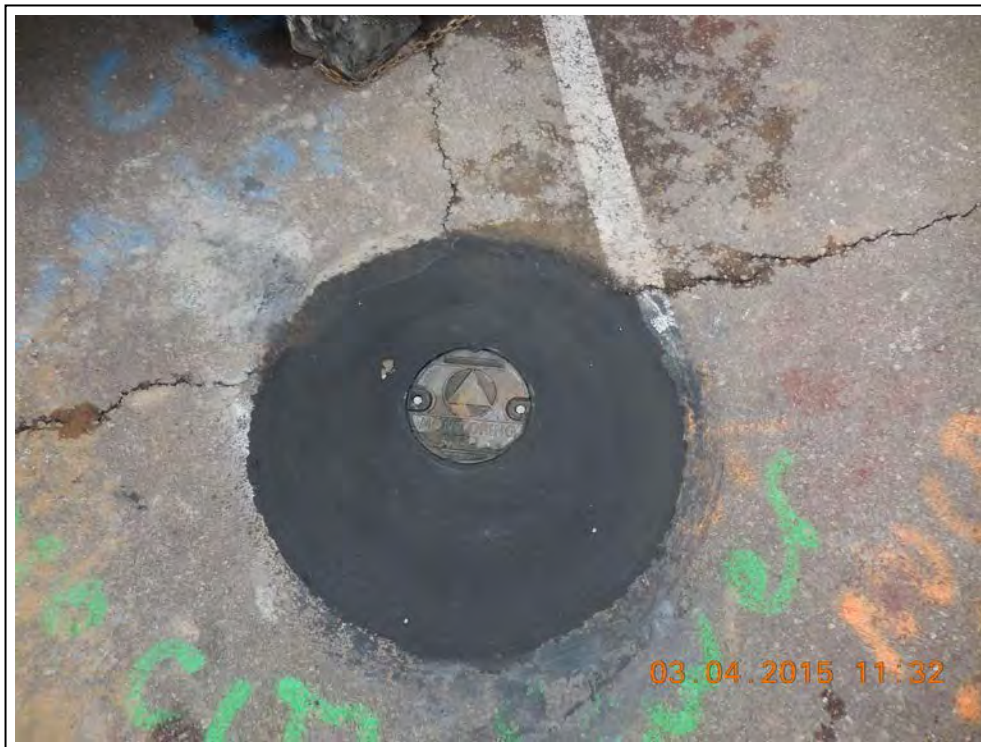
7. Surface completion of MW-10.
