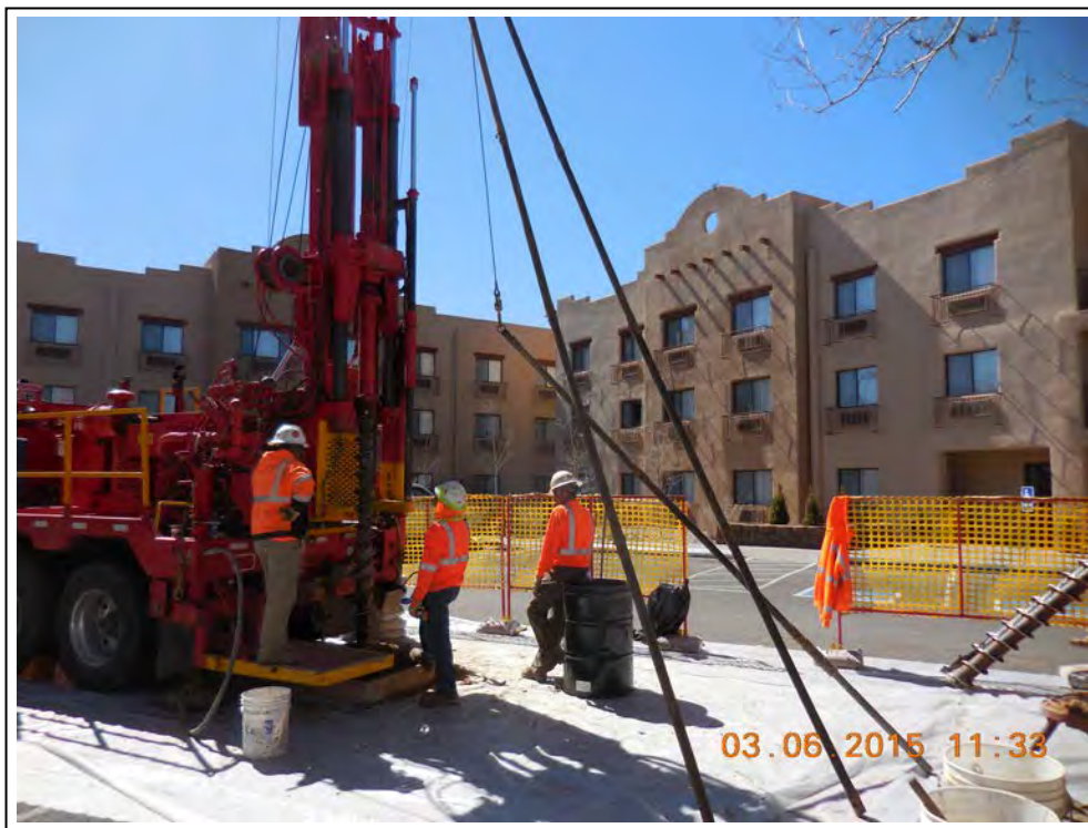
19. Drilling monitor well MW-12.
