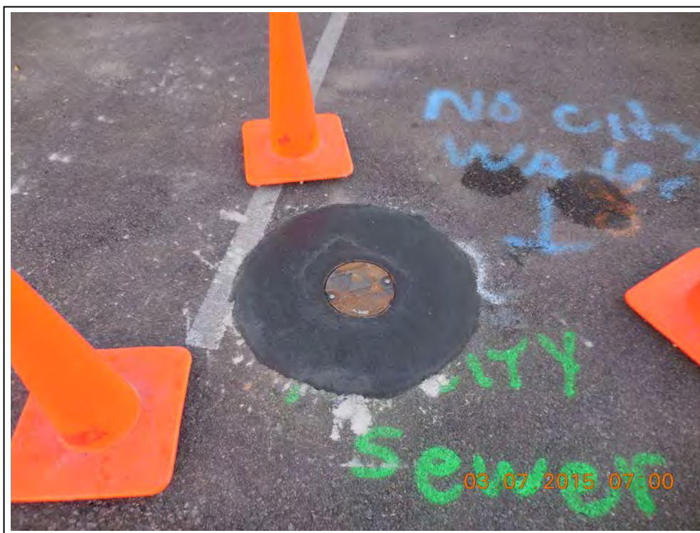
20. Surface completion of MW-12.
