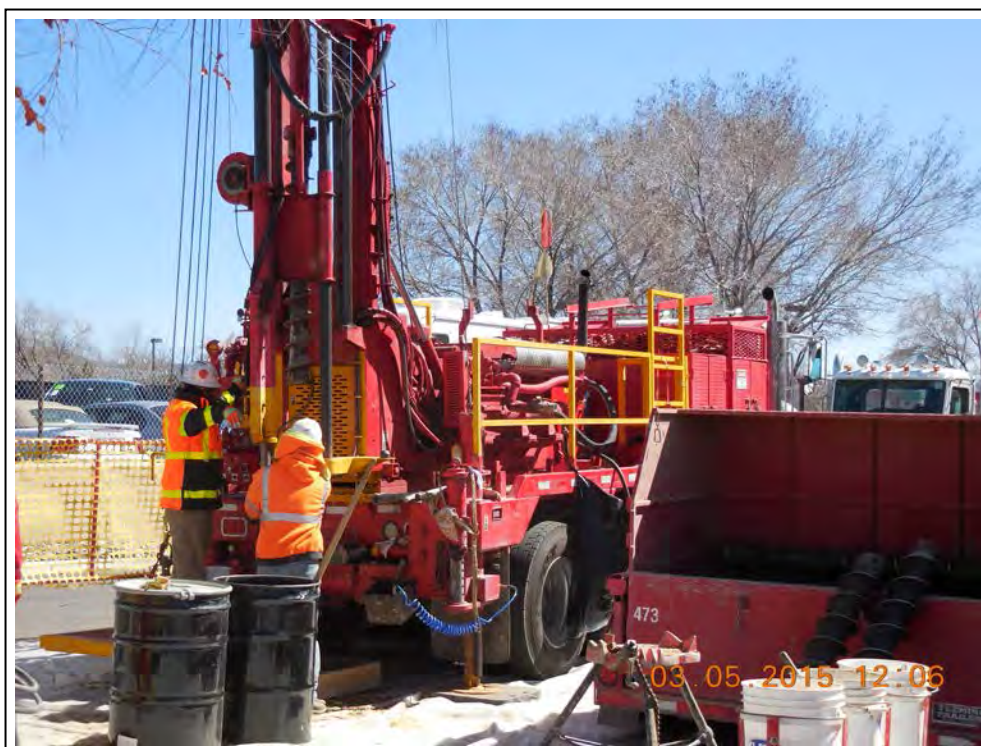
14. Drilling monitor well MW-11.
