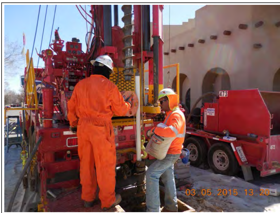
16. Installation of filter pack at MW-11.
