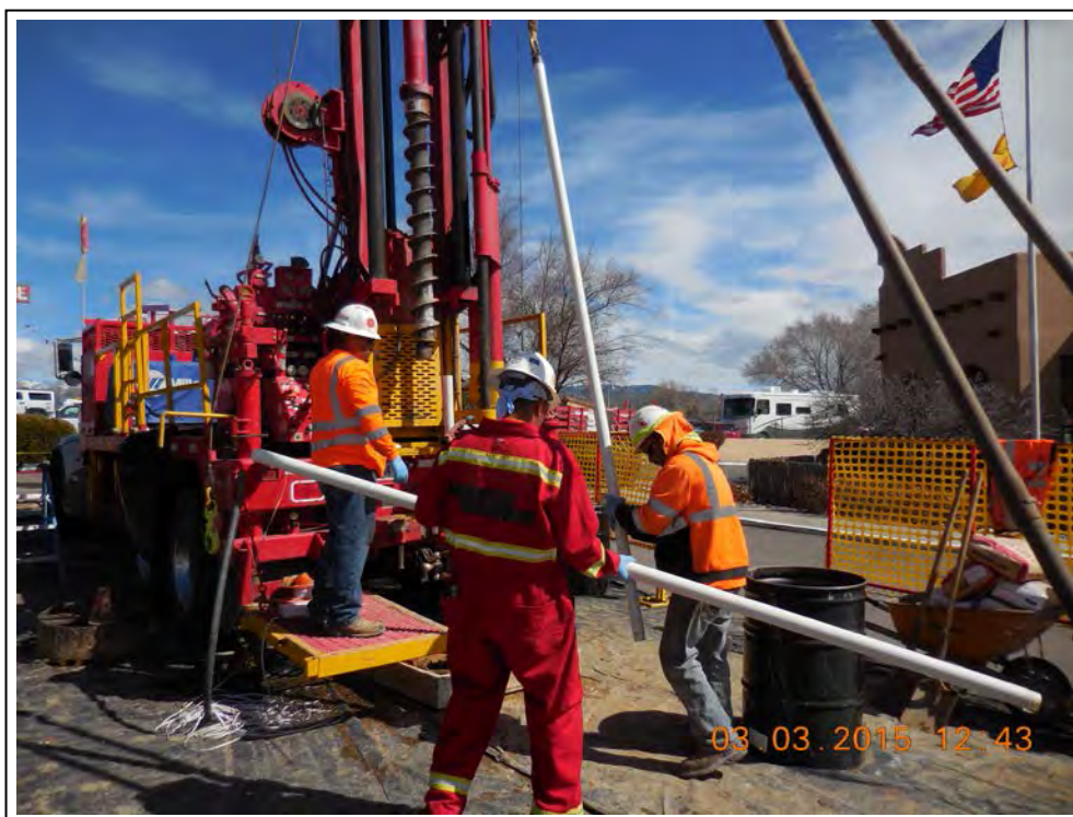
4. Installation of well casing at MW-10.
