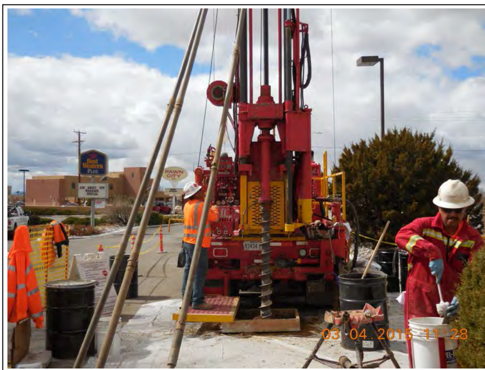
10. Drilling monitor well MW-9 and decontamination of split spoon sampler.
