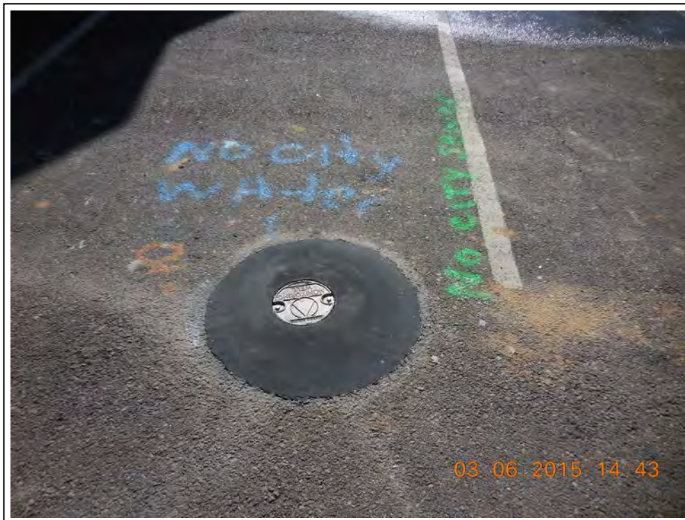
17. Surface completion of MW-11.
