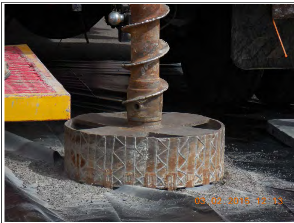
2. Removal of surface asphalt at MW-10.
