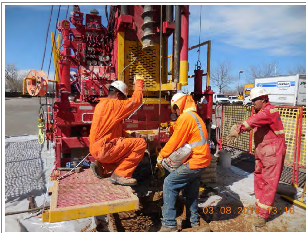
27. Installation of filter pack at MW-13.
