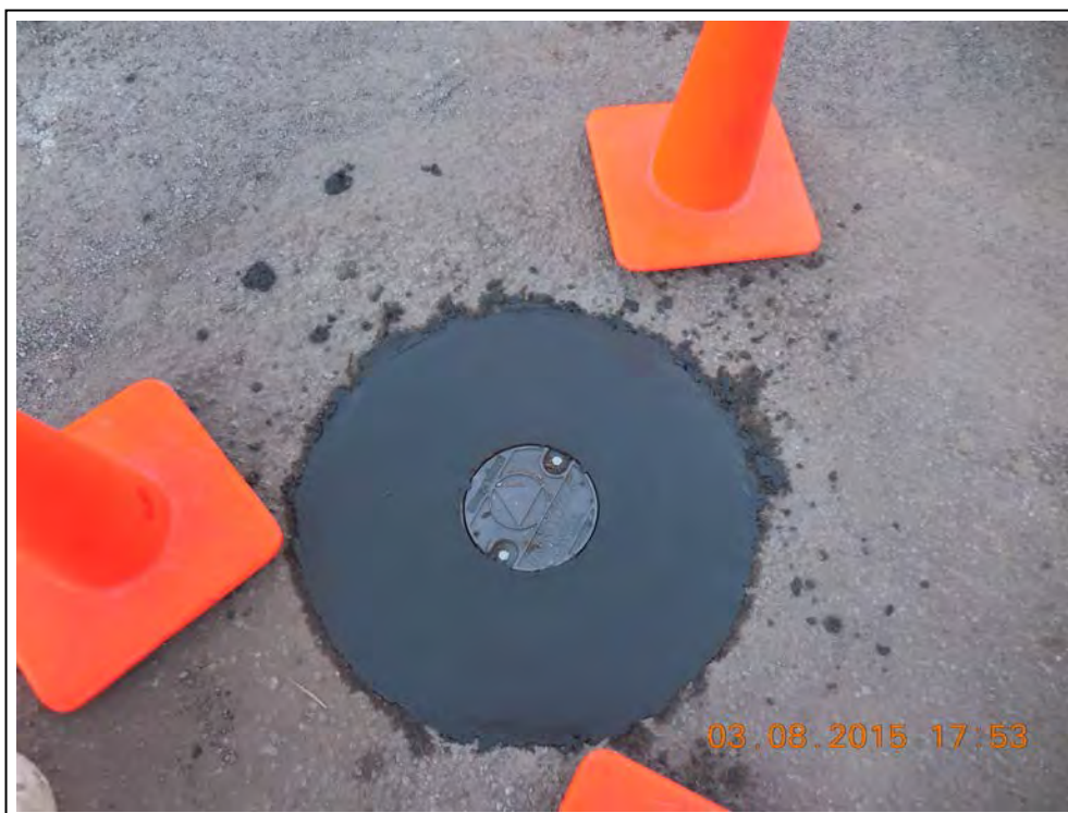
28. Surface completion of MW-13.
