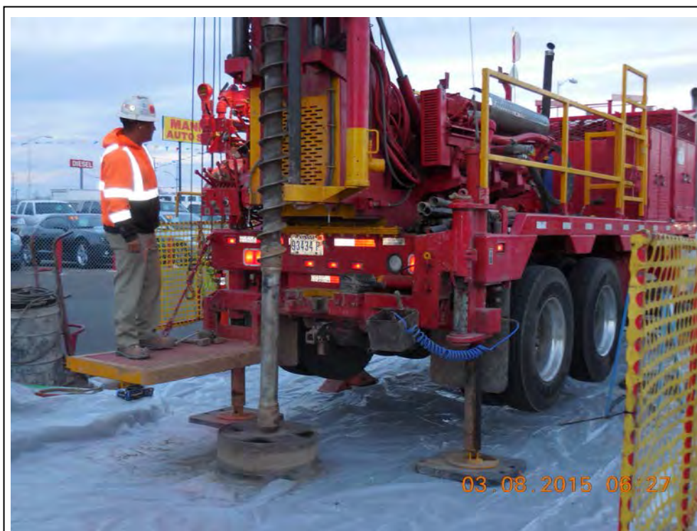
26. Removal of surface asphalt at MW-13.
