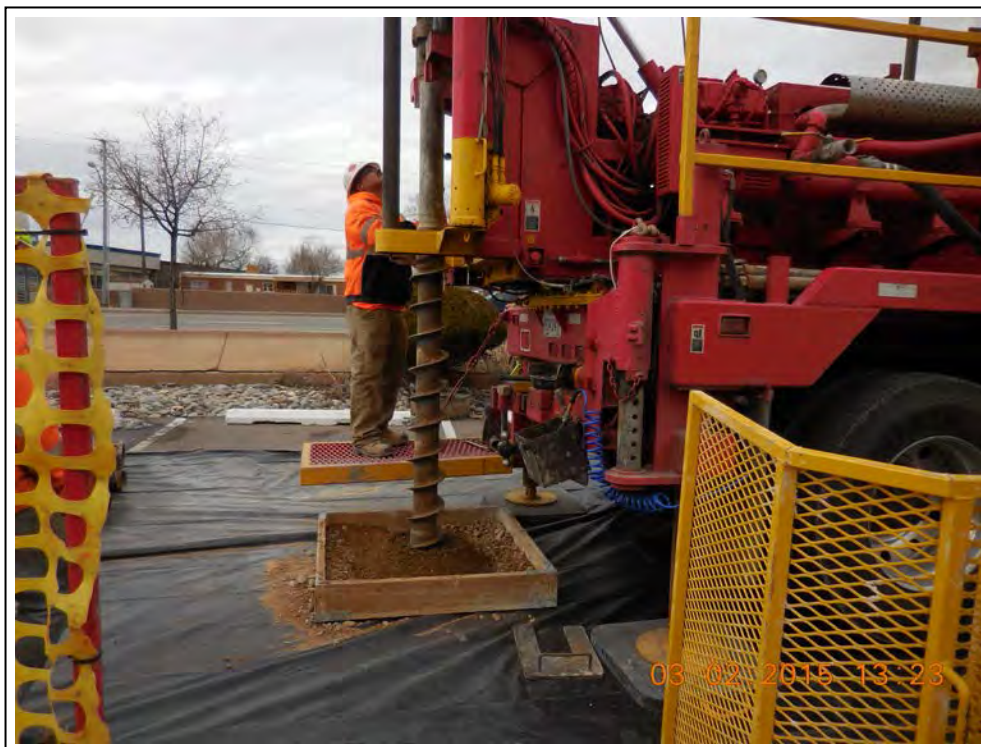
3. Drilling monitor well MW-10.
