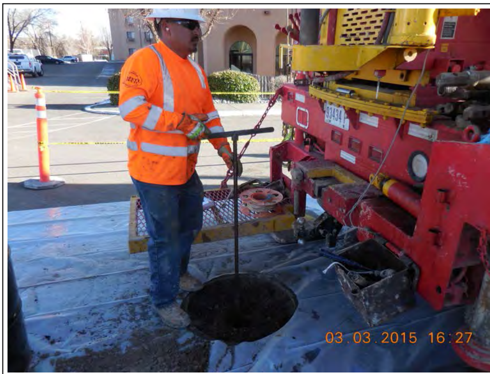
9. Hand auger clearance at MW-9.
