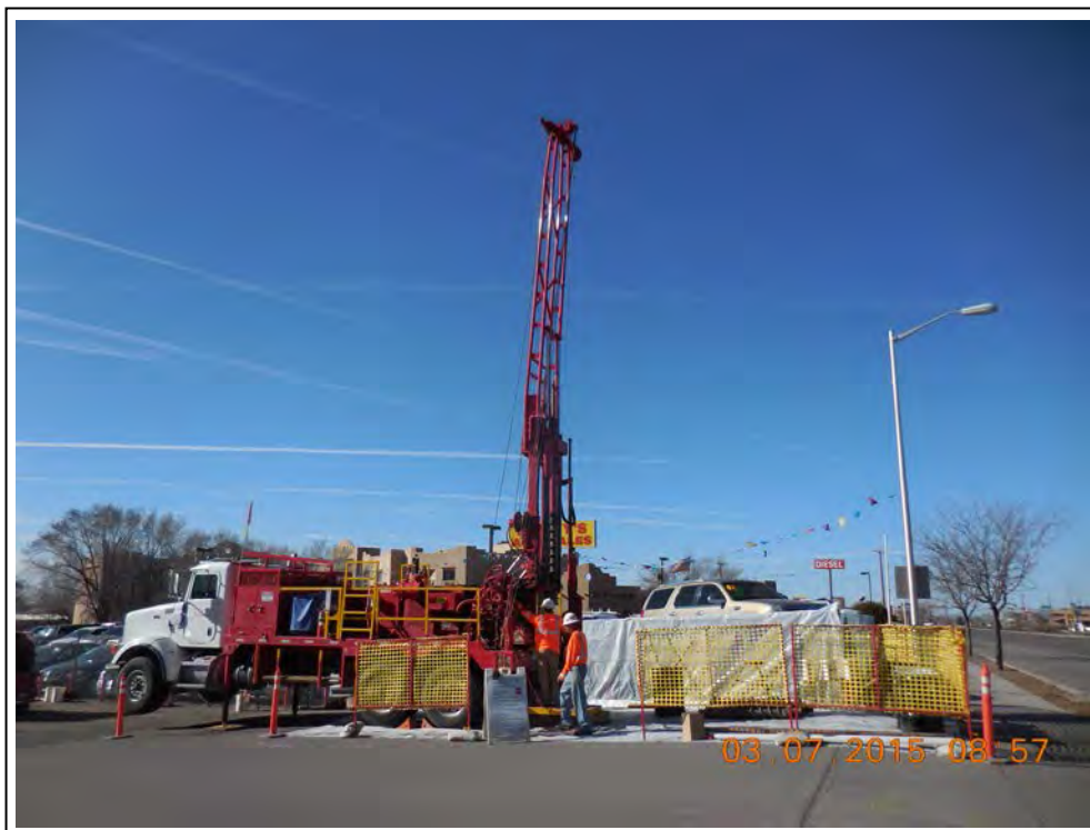
21. CME-85 rig and exclusion zone at MW-14.
