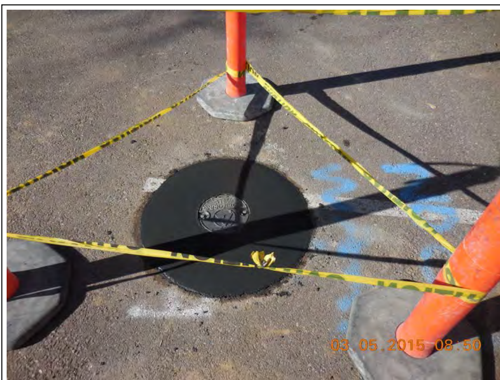
12. Surface completion of MW-9.
