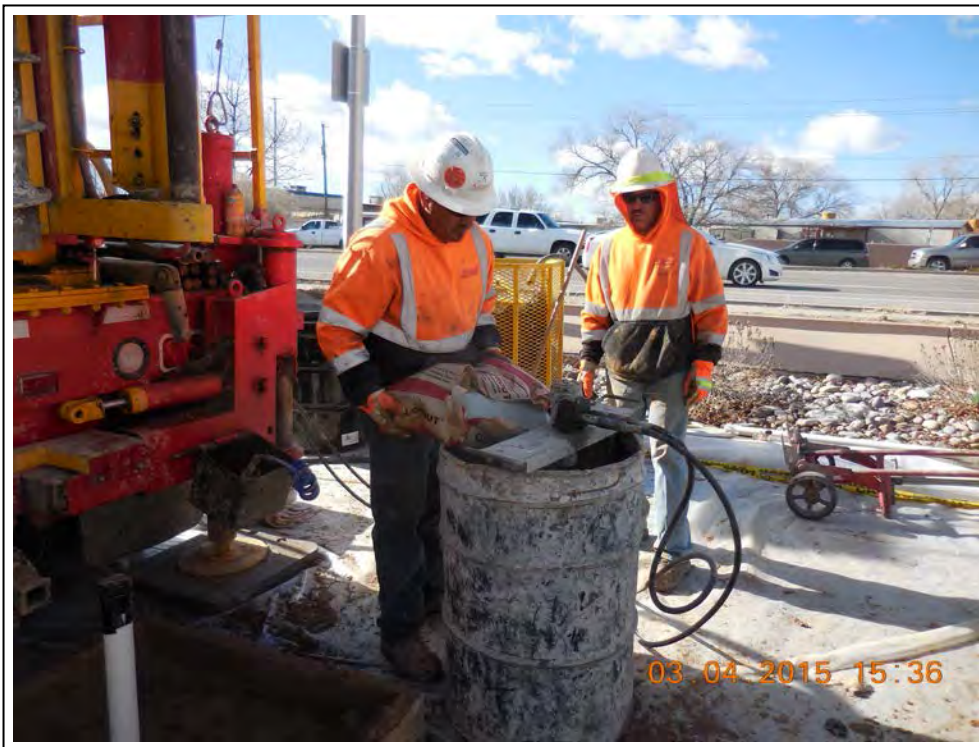
11. Grout mixing at MW-9.
