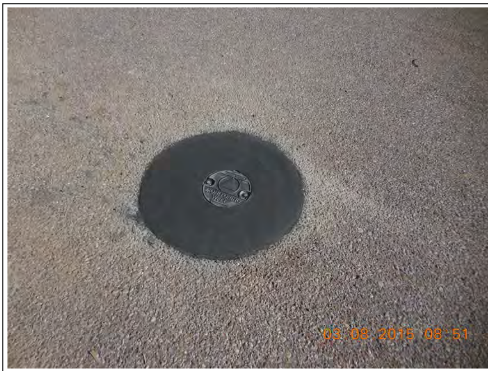
25. Surface completion of MW-14.
