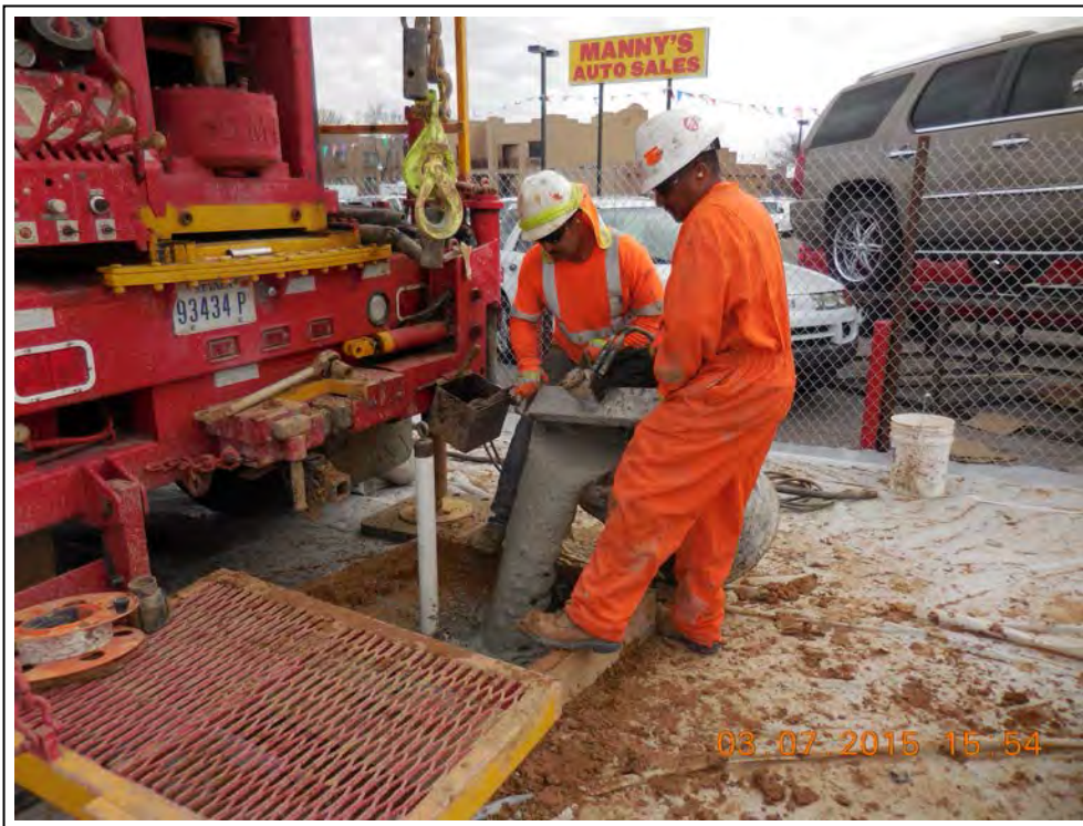
23. Installation of grout at MW-14.
