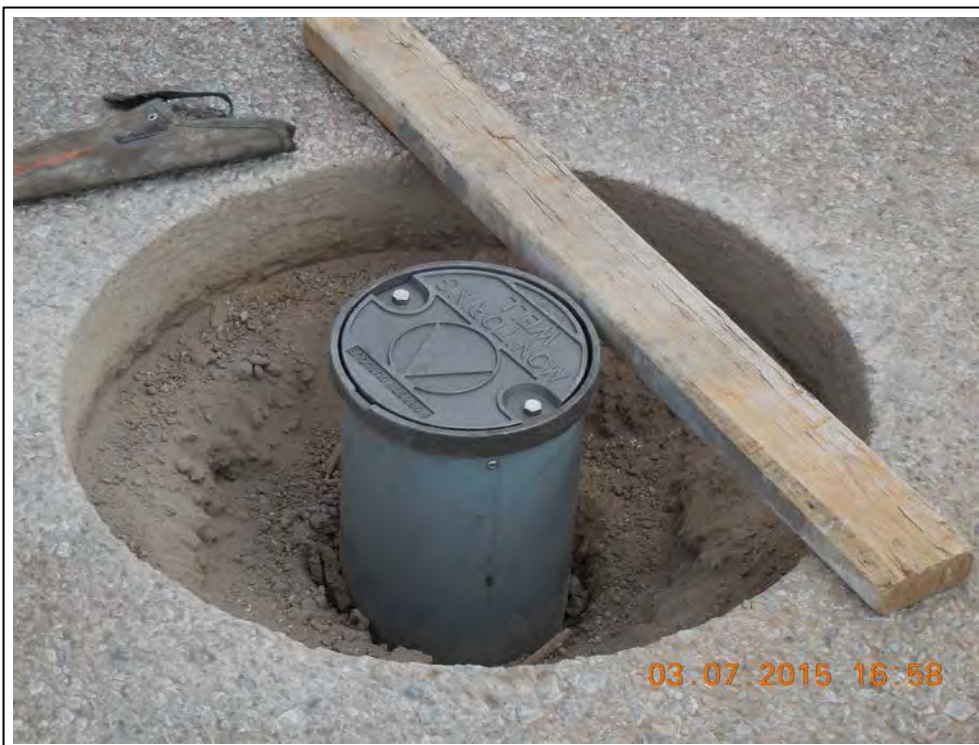
24. Installation of flush-mount, traffic-grade vault at MW-14.
