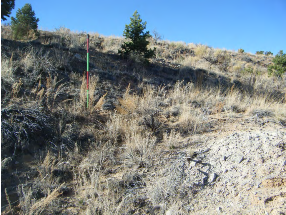
Photo 9-Looking southwest at PilePly-2.
