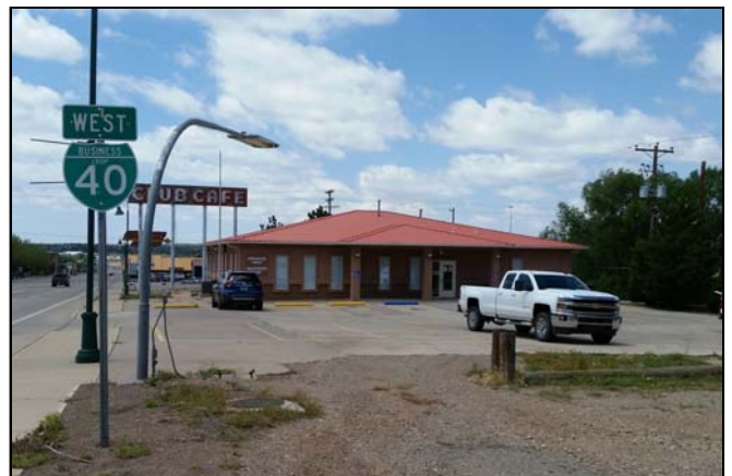
Picture 12 – Overall view of Site from the southeast corner.
