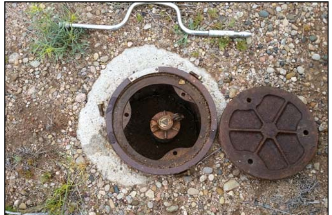
Picture 10 - Looking down MW-2A. Well vault in good condition.
