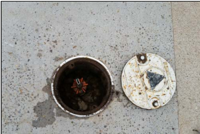
Picture 9 – Looking down MW-1A. Well vault in good condition.
