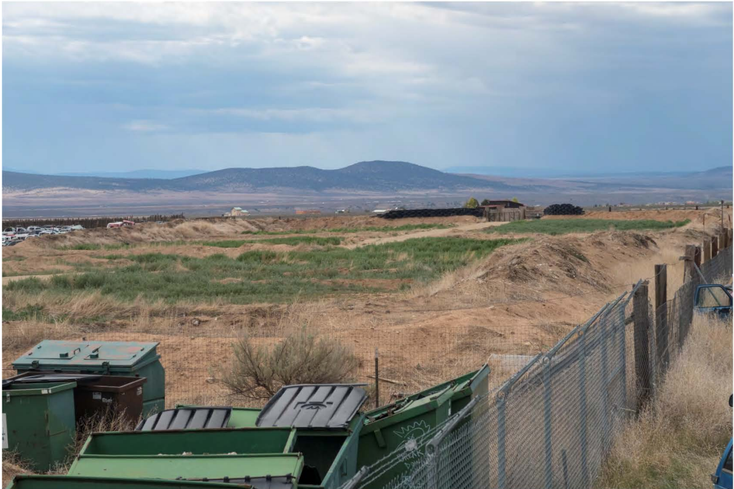
Figure 7. The septic system 7/2018.
