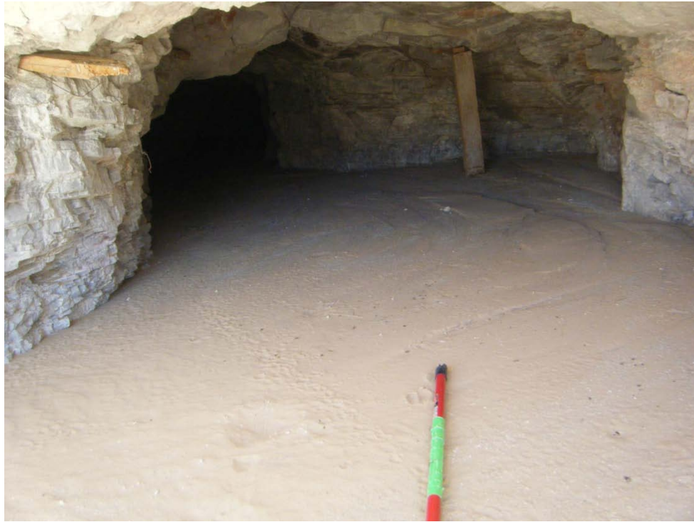
Photo 23-Looking northwest into Adit-6 (Blackhawk/Bunney claims).
