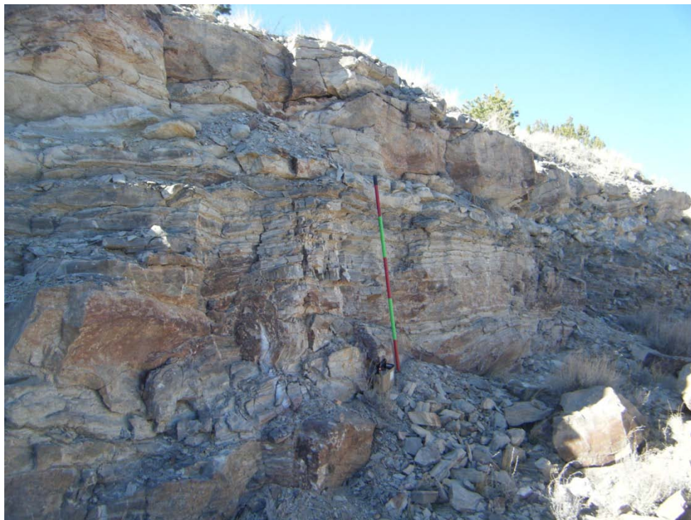
Photo 58-Looking southwest at rock face in Pit-9 (Red Bluff No. 7 claim).
