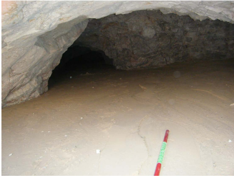
Photo 31-View into interior of Adit-8 (Blackhawk/Bunney claims).
