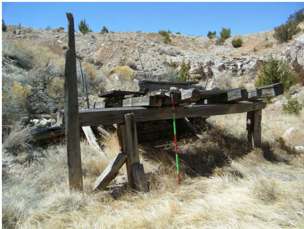
Photo 24-Looking west at old mine structure (StrucPly-1; Blackhawk/Bunney claims).
