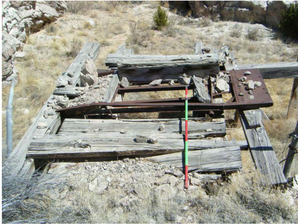
Photo 25-Looking east at StrucPly-1 (Blackhawk/Bunney claims).
