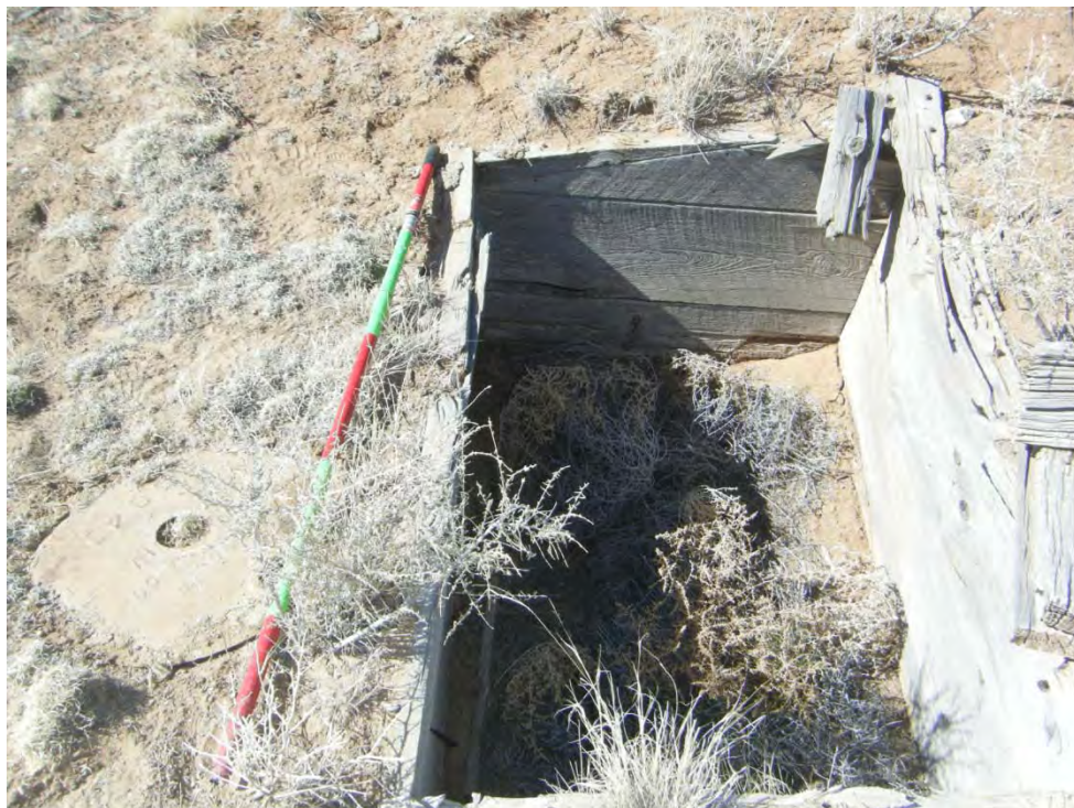
Photo 68-A wooden structure sunk into the ground (StrucPly-2; Red Bluff No. 7 claim).
