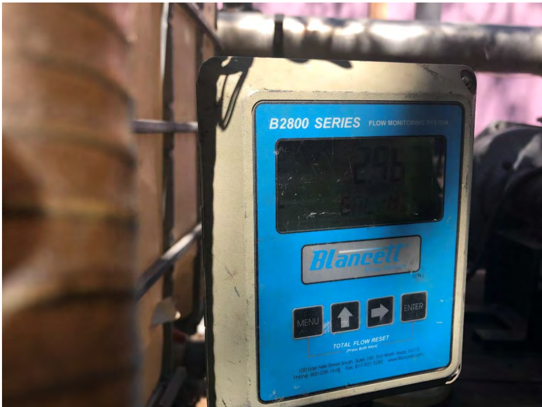
Photograph 2: Fluids flow meter/totalizer
