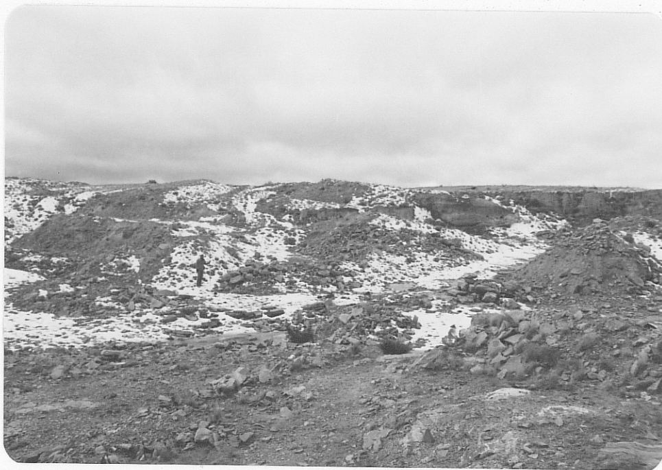
Photo (d) Side workings off the area shown in (c); extensively worked pit with gamma levels ranging up to 2,800 cps. Note person for scale.
