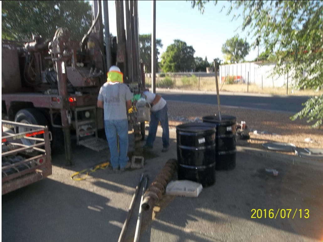
Photograph No. 9 Description: Placing filter pack around well screen in MW-17.
