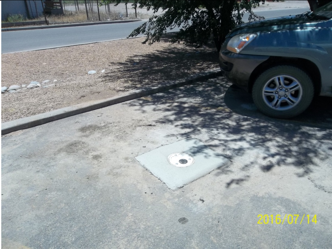
Photograph No. 13 Description: Completed well, MW-17.
