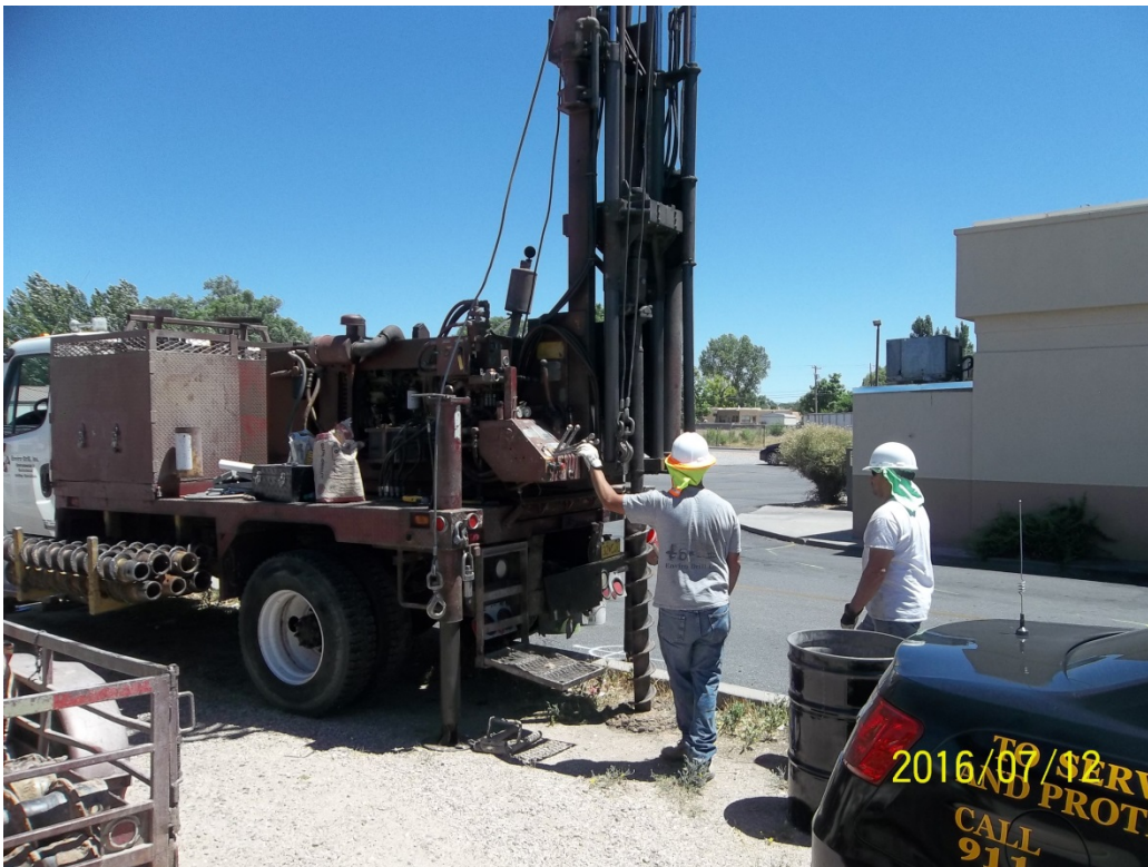
Photograph No. 8 Description: Drilling MW-18.
