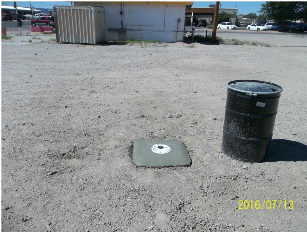
Photograph No. 12 Description: Completed well, MW-16.
