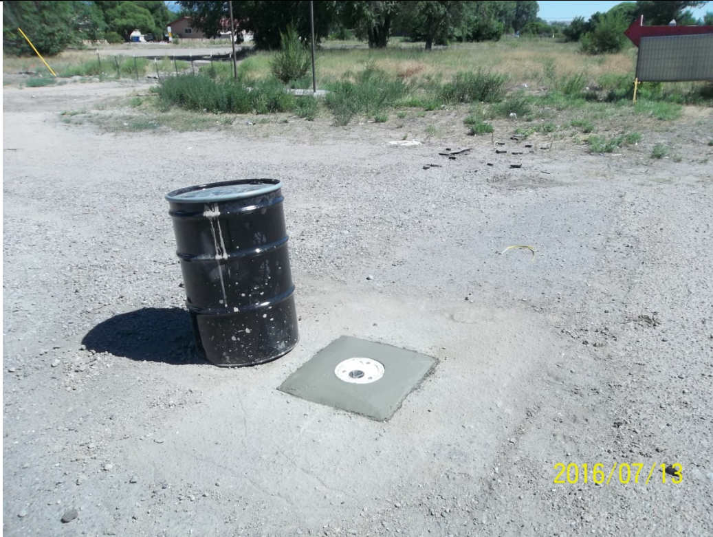
Photograph No. 11 Description: Completed well, MW-15.
