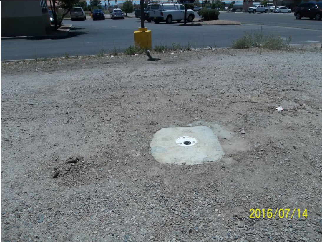
Photograph No. 15 Description: Completed well, MW-19.
