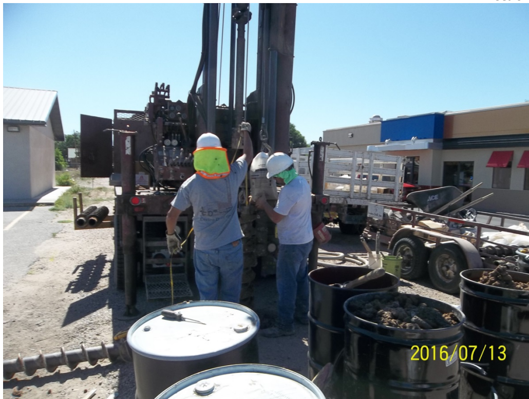
Photograph No. 10 Description: Placing filter pack around well screen in MW-19.
