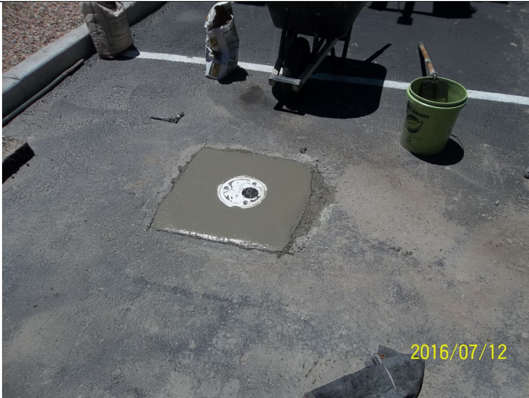
Photograph No. 7 Description: Completed well, MW-20.
