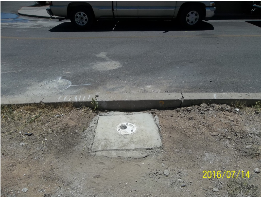
Photograph No. 14 Description: Completed well, MW-18.
