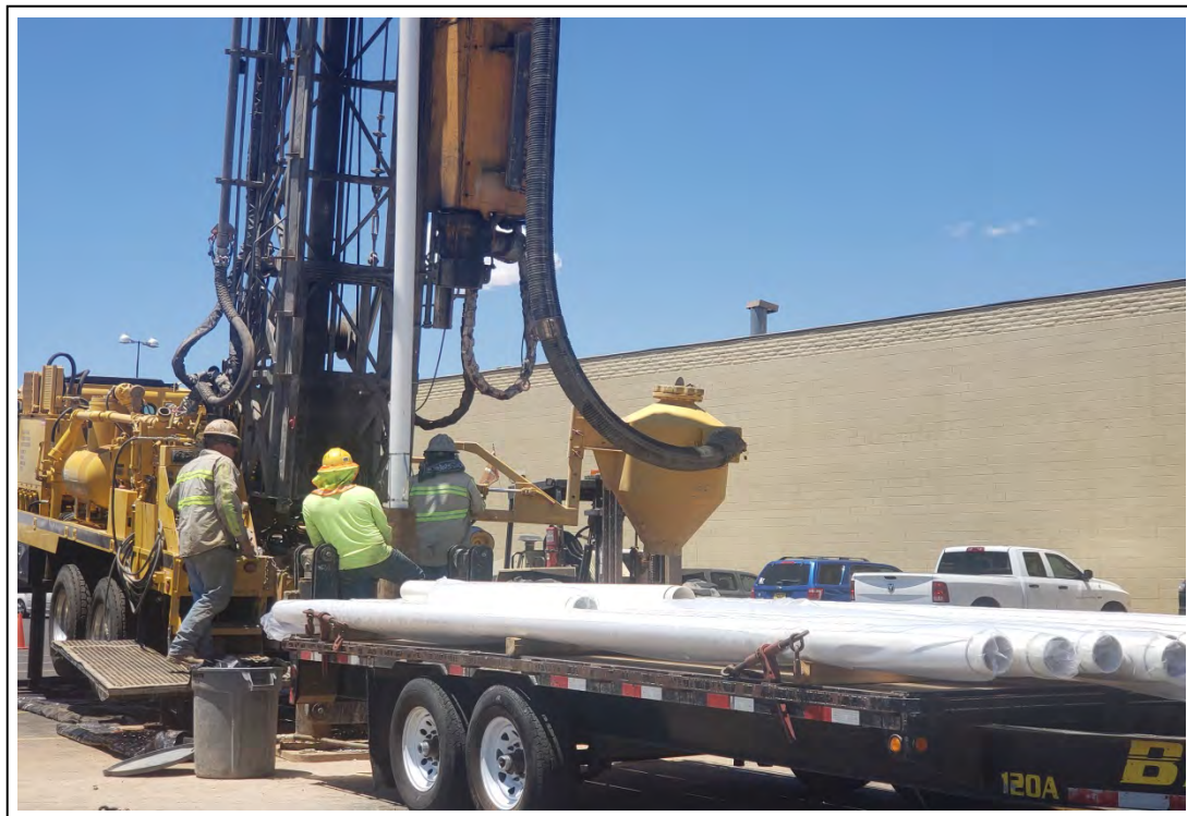
6. Installing centralizers in MW-16, view to the northwest.
