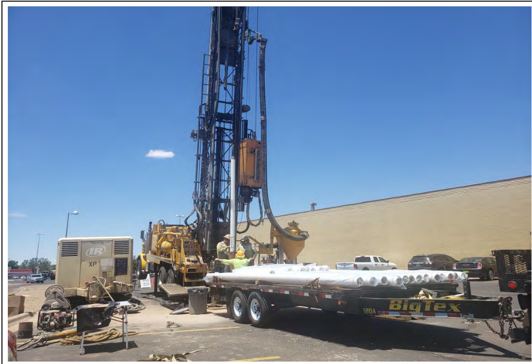
5. Installing casing in MW-16, view to the northwest.
