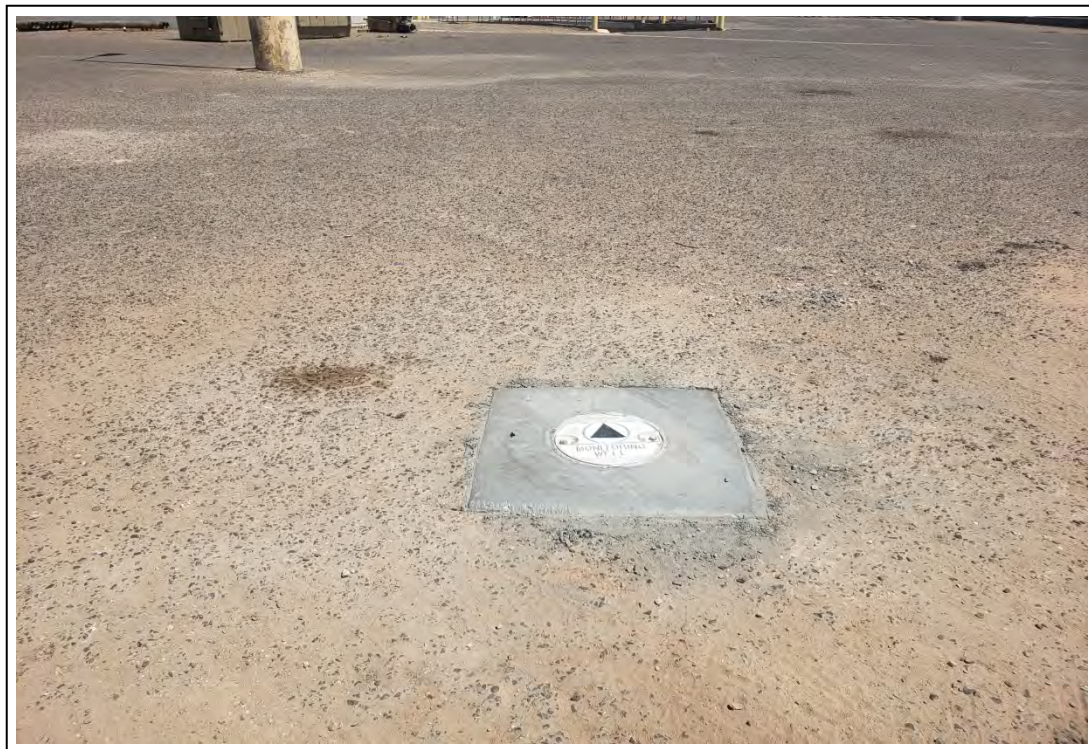
16. Completed monitor well MW-17, view to the north.
