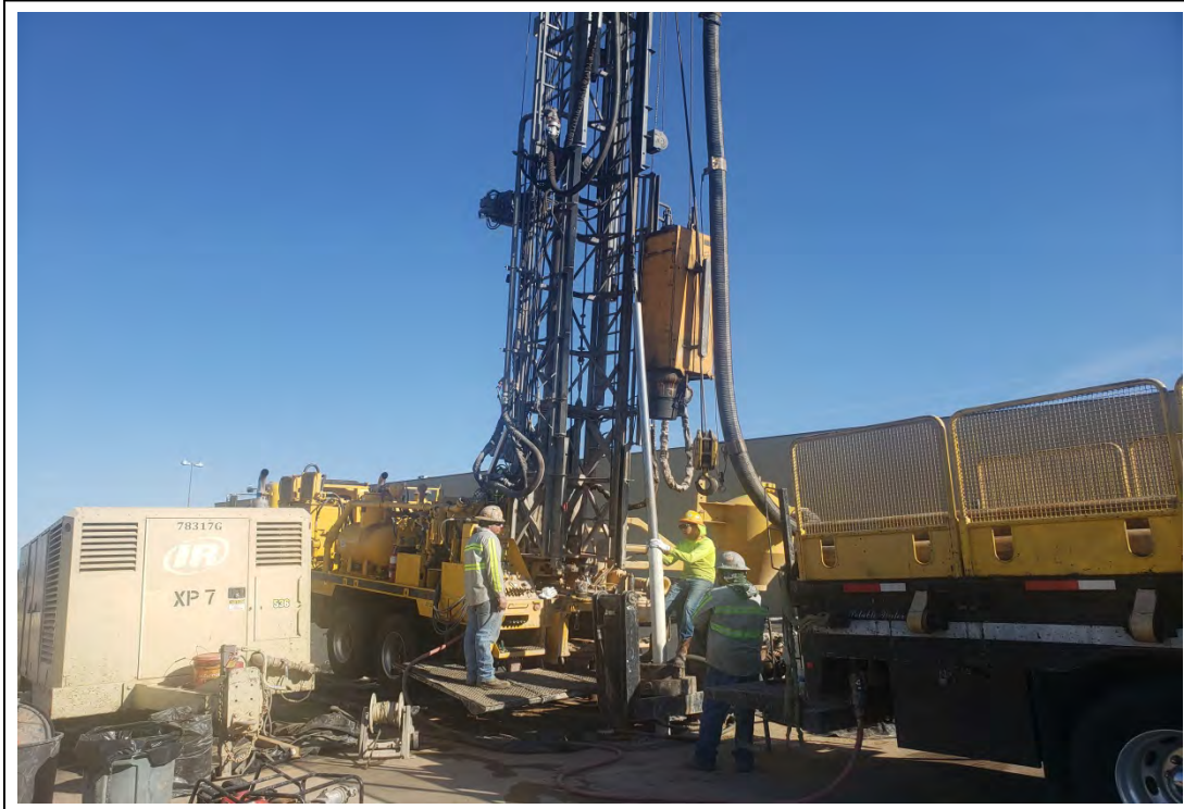
9. Deploying dummy pipe in MW-16, view to the northwest.
