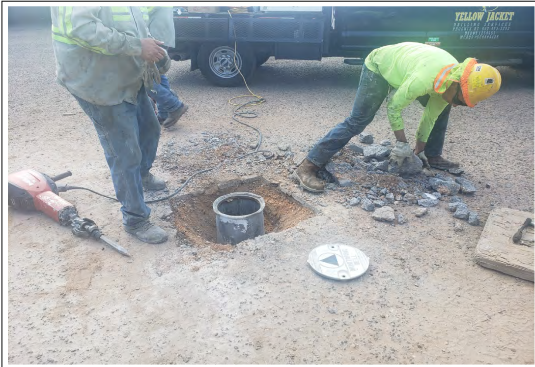
3. Installing surface completion at MW-17, view to the northwest.
