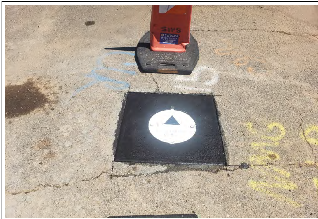
14. Completed monitor well MW-15, view to the north.
