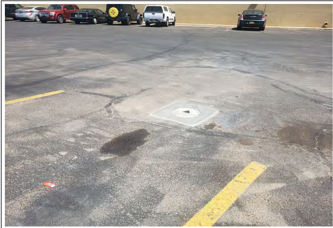
15. Completed monitor well MW-16, view to the northwest.
