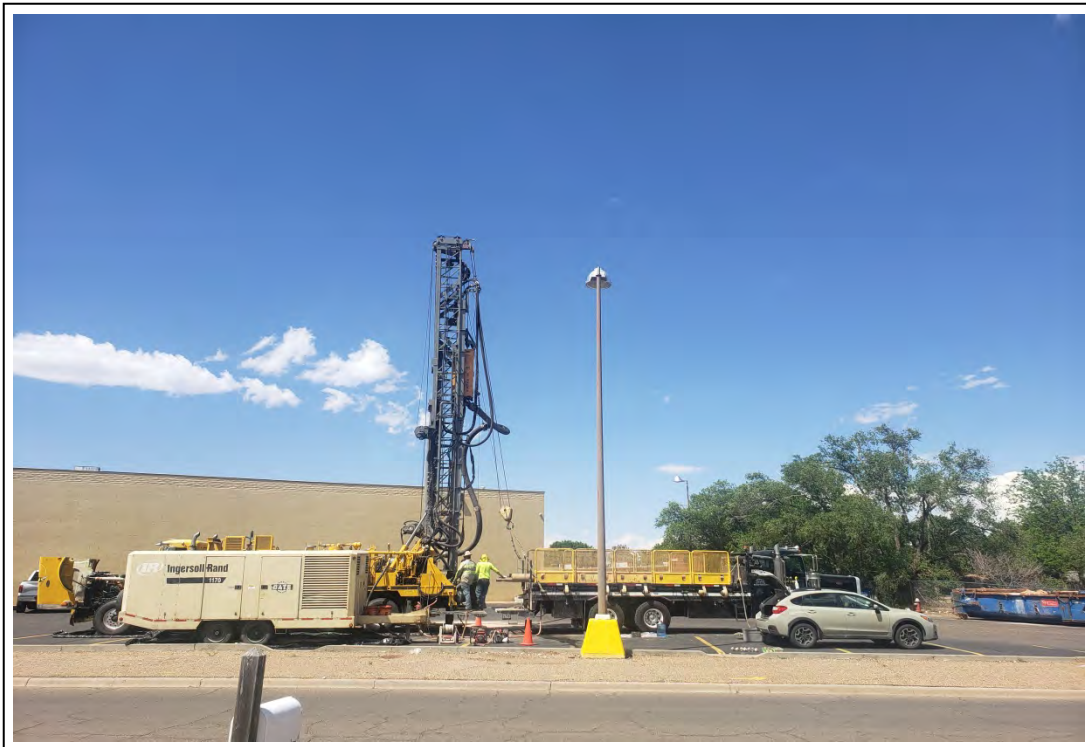
4. Drilling MW-16, view to the north.
