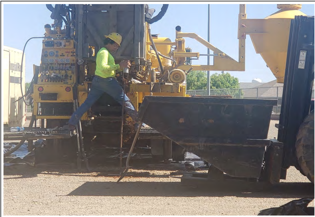
2. Hand-augering the first few feet of MW-17, view to the north.
