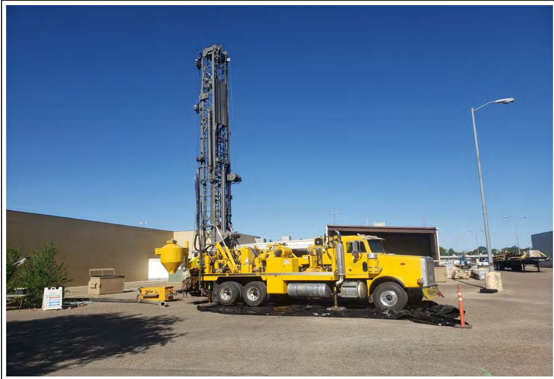
1. Setting up to drill MW-17, view to the west.
