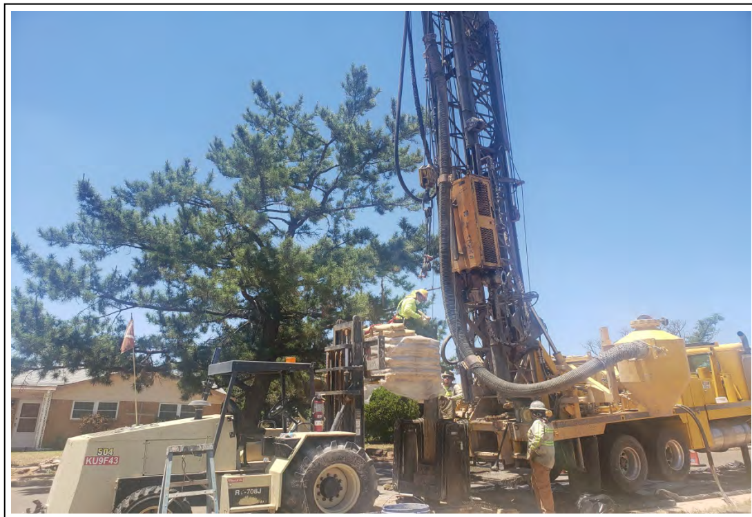
12. Installing sand filter pack in MW-15, view to the west.
