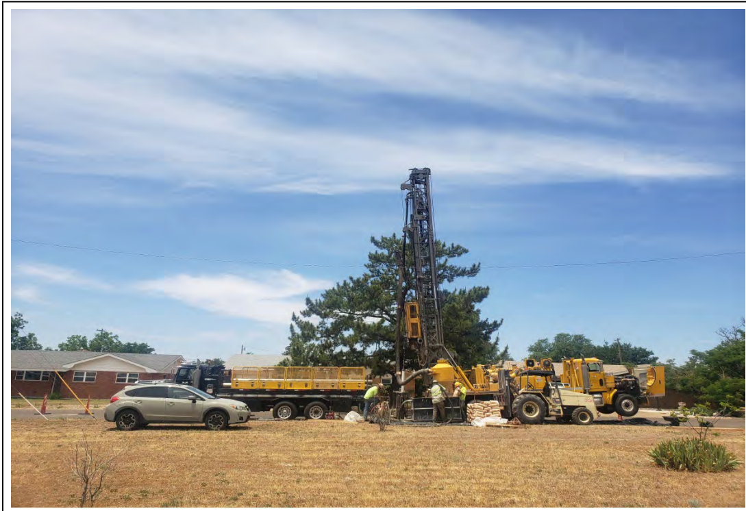
13. Grouting MW-15, view to the west.
