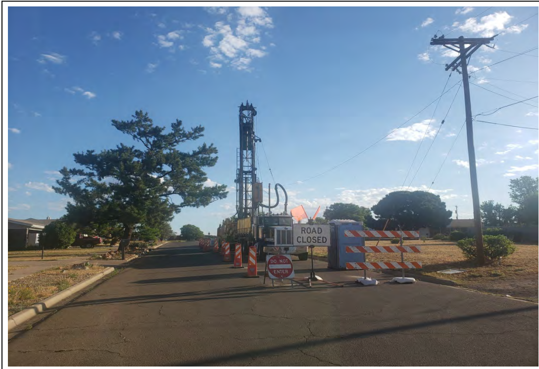
11. Traffic control for MW-15, view to the north.
