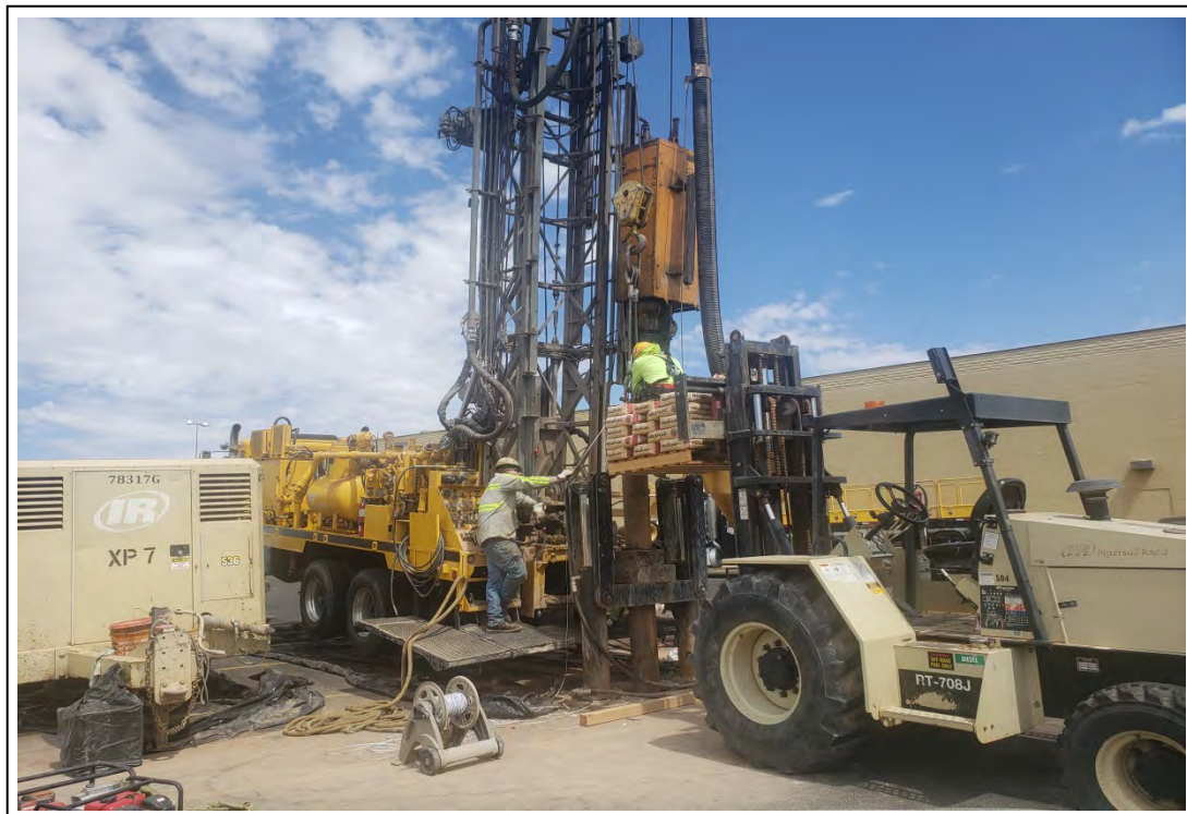
8. Installing bentonite seal in MW-16, view to the northwest.
