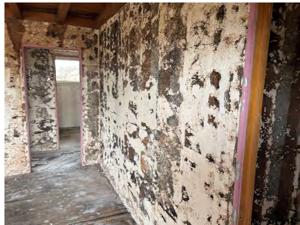
Waste Cleaned Out of House after Abatement Completion
