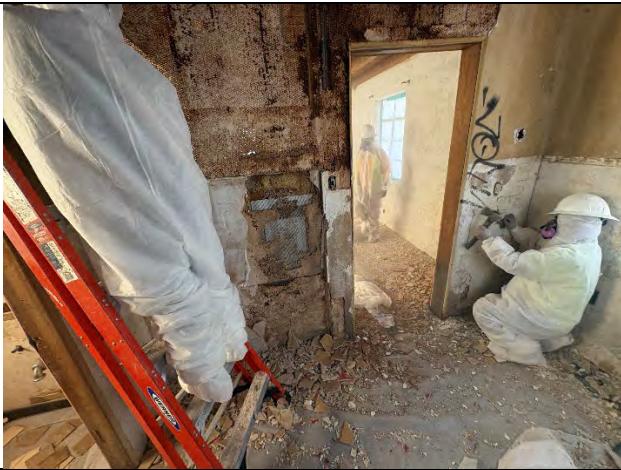
Gancor Three Workers Using Wet Methods
