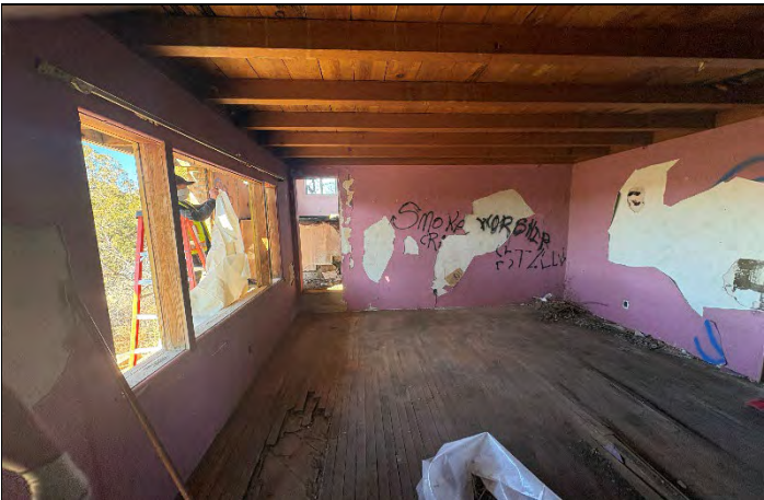
Inside of House Before Abatement
