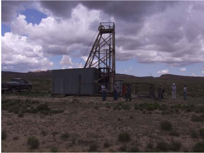
P1: Operational hoist over mineshaft
