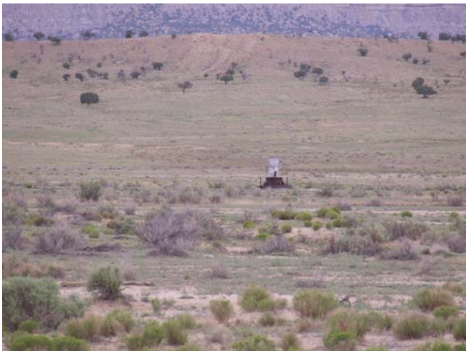
P3: A ventilation shaft distant from main shaft
