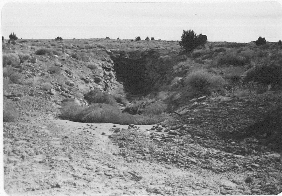
Photo A - looking south at pit entrance to collapsed adit.
